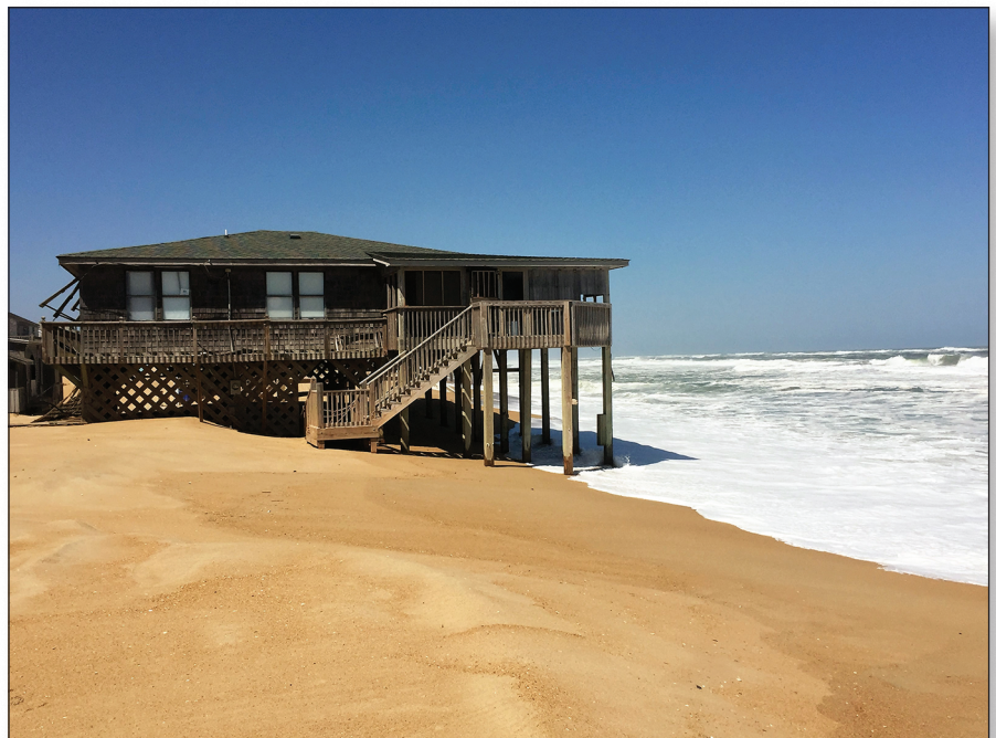
Figure 4. A home in the surf on the Outer Banks, North Carolina. (Credit: Jonathan Phinney/USFWS).
