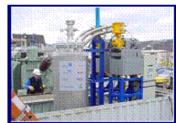
CURL 10 Fault Current Limiter
