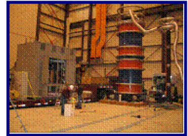
Testing of Zenergy's FCL device
