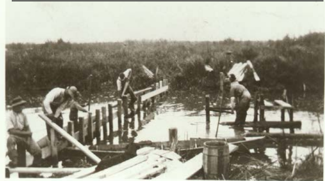
Horicon Shooting Club members plugging the ditch
