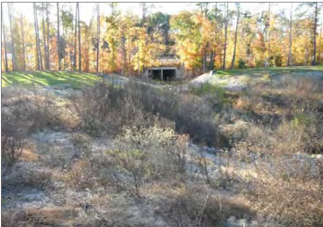
Figure 8. Tributary and Culvert under US 69 in Western Portion of APE (Facing NW)
