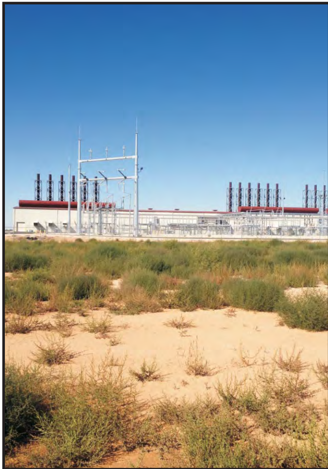
PHOTO 1 View of Antelope Station expansion area looking towards existing Antelope Facility
