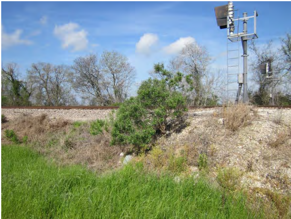
Photograph 14. Railroad ROW along existing pipeline ROW
