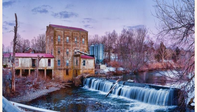
The Weisenberger Mill, a Civil War-era family-owned and operated mill in Kentucky, used Department of Energy funding to install a generator and power electronics. The new system utilizes water flowing through the turbines more efficiently, generating enough power to run the mill when it is grinding.
