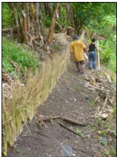
Before: Installation of a Vegetative Barrier.
