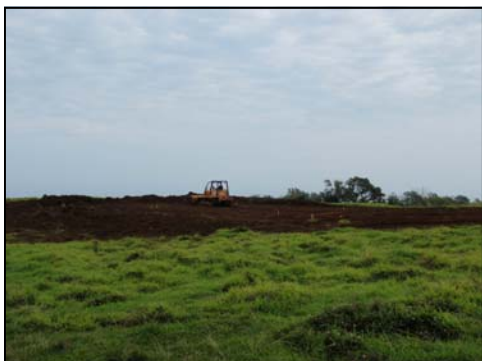
A pond is built as part of a livestock watering system. This practice, along with pipeline, troughs, fencing and noxious weed control measures, facilitates the implementation of a rotational grazing system to address a variety of resource concerns.
