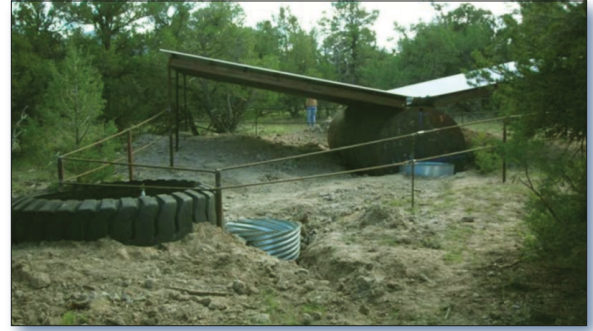
Figure 3. This completed livestock "trick tank," an alternative water source installed in an upland area, reduces grazing pressure on the riparian corridor.
