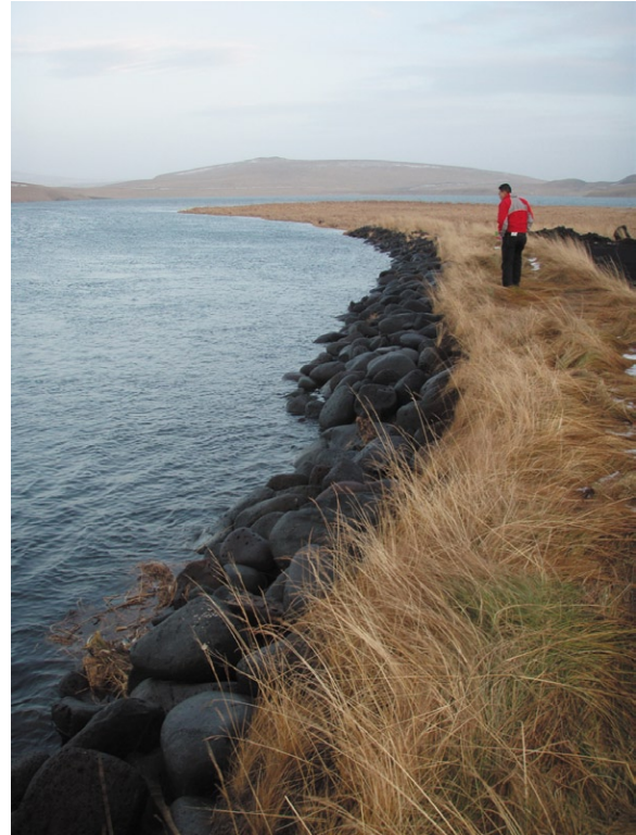
Figure 1. The Salt Lagoon Diesel Seep area after NOAA removed contaminated soil and restored the St. Paul Salt Channel shoreline.
