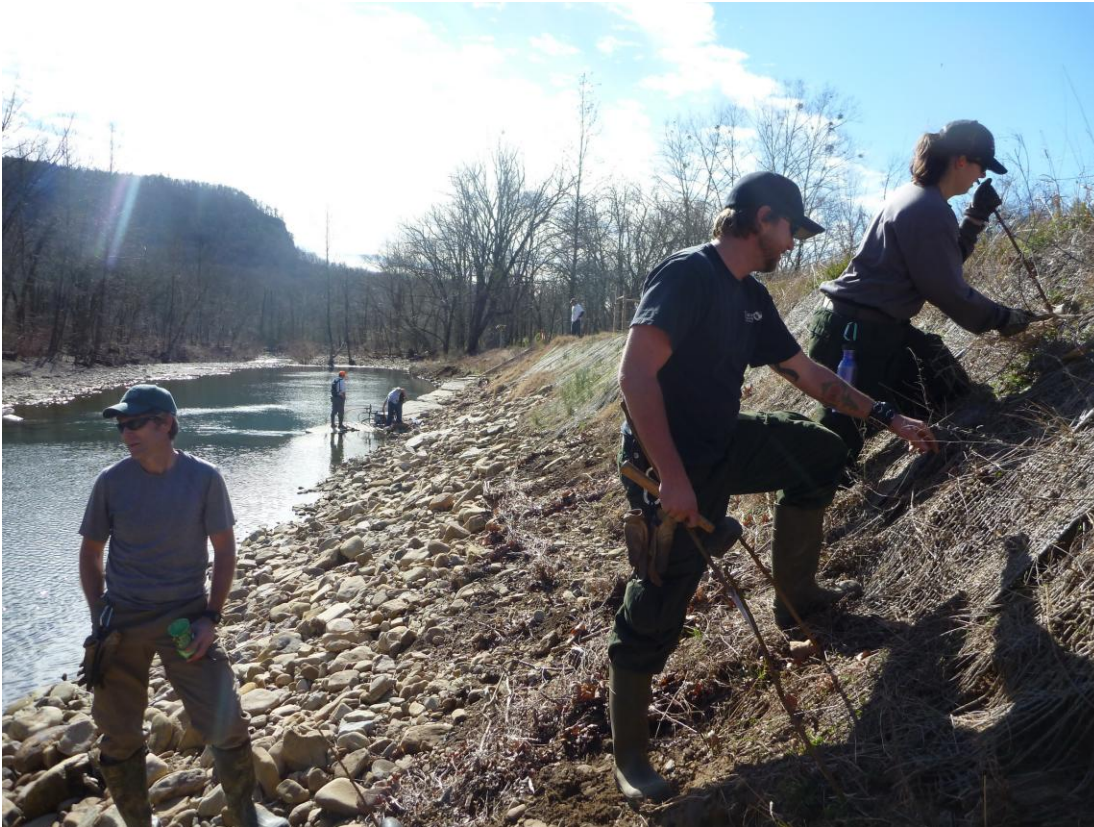
Bank stabilization work: Upper Little Red River watershed
