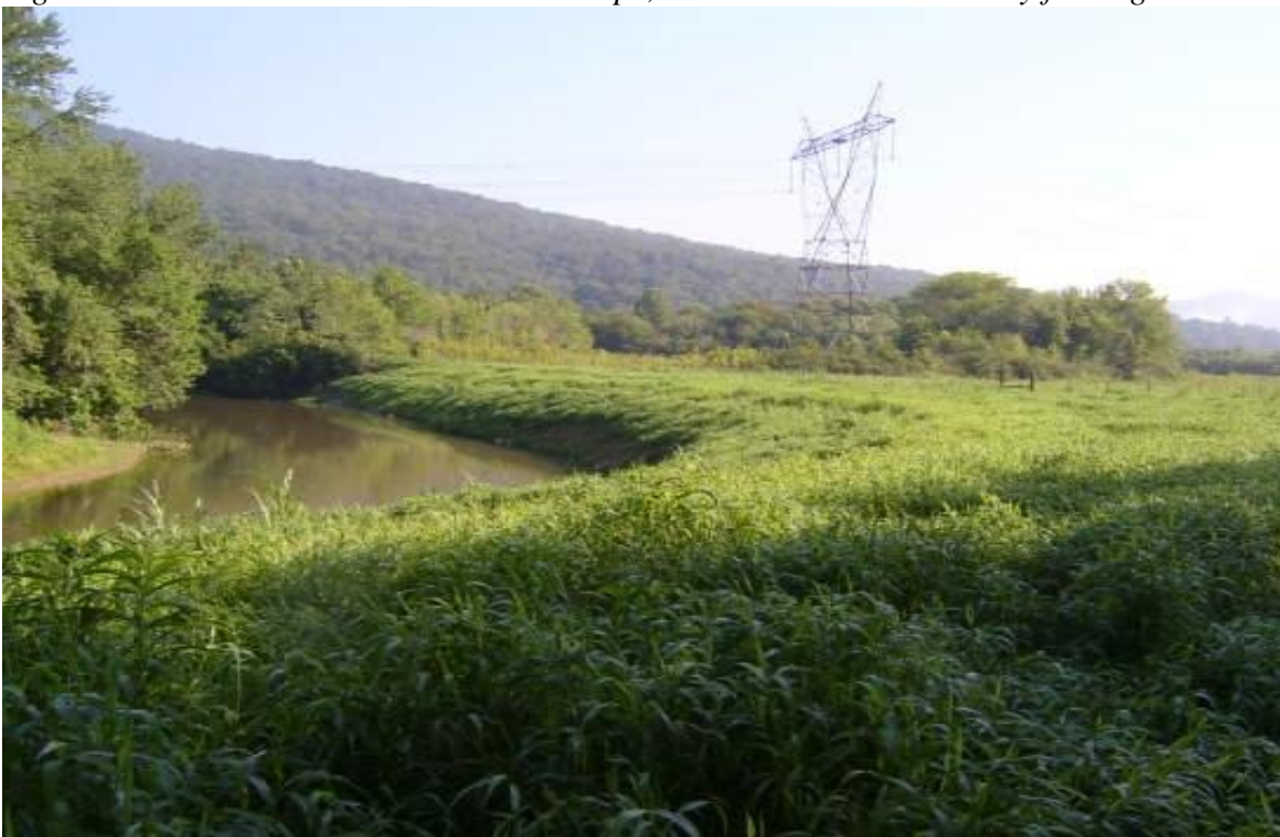
Paint Rock River, AL: After project: Re-contoured bank with rock at the toe of the slope, vegetated erosion control blanket on the slope, and livestock exclusionary fencing.
