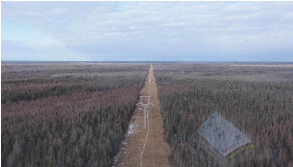
Figure 6.10-2. Aerial View of Existing 500kV Transmission Line in Forested Setting
