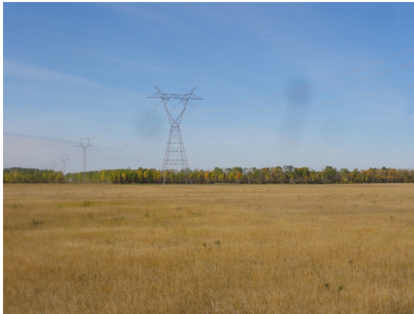
Figure 6.10-1. View of Existing 500kV Transmission Line in Agricultural Setting
