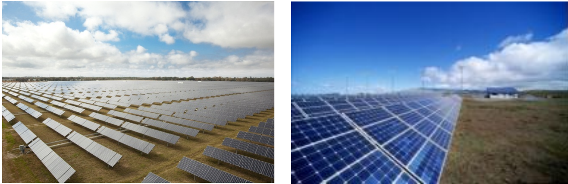
Figure 3. Mono-crystalline (left) and multi-crystalline (right) solar panels. Photos from (left) SunPower Corporation, NREL 23816 and (right) SunPower, NREL 13823
