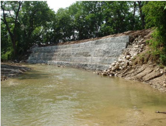
Figure 3 – Streambank Protection: Gabion Baskets with shotcrete facing
