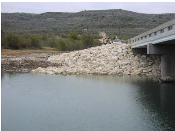
Figure 11 – Bridge abutment stabilization: Rock riprap armor
