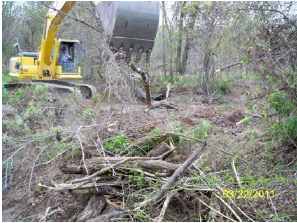
Figure 13 – Woody debris removal in ephemeral stream channel
