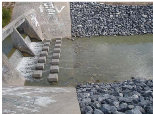
Figure 17 – Drainage Ditch Stabilization: Rock armor of concrete weir
