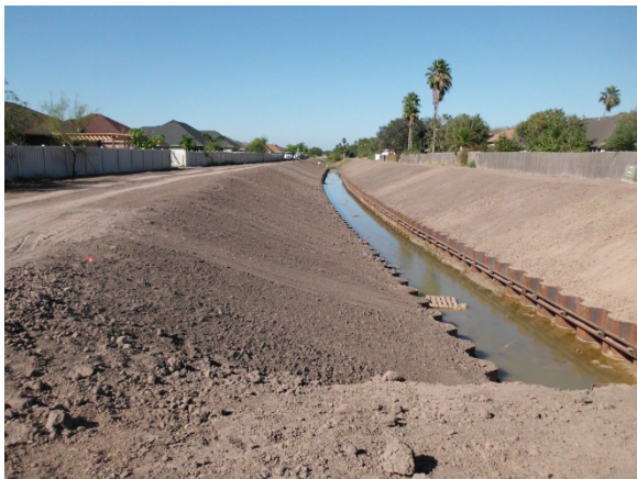
Figure 16 – Drainage Ditch Stabilization: Steel sheet piling and bank shaping
