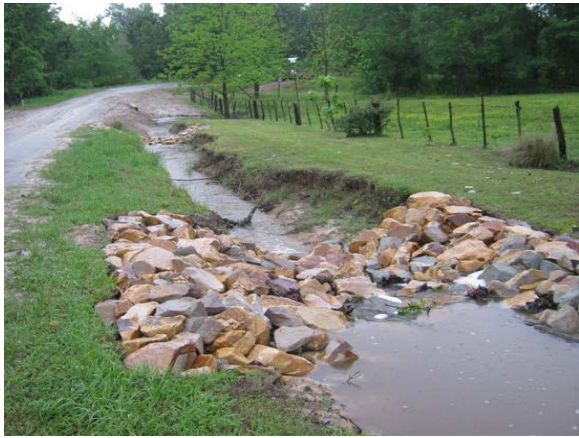
Figure 9 – Ditch Stabilization: Rock riprap check dams
