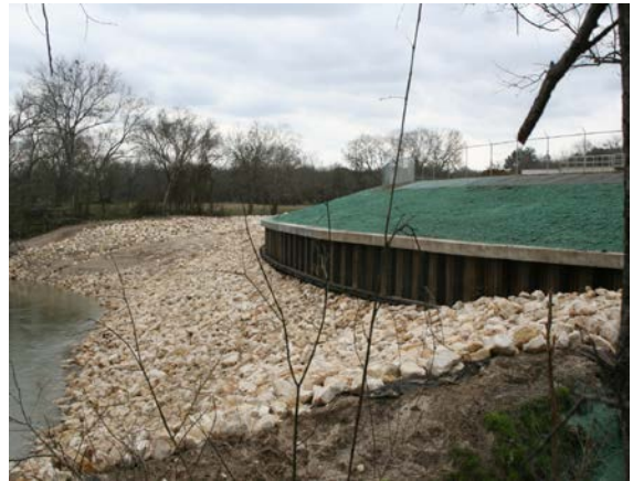
Figure 4 – Streambank Protection: Steel sheet piling with rock armor
