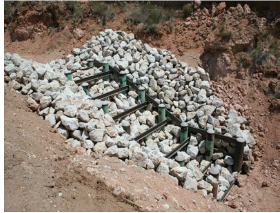
Figure 8 – Ditch Stabilization: Rock filled steel piling and rails
