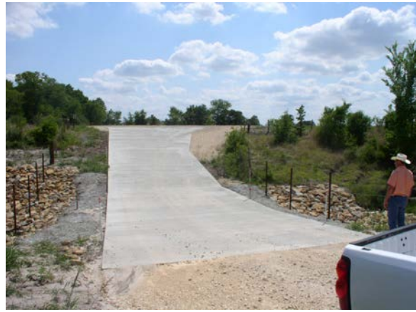
Figure 10 – Low water crossing: Concrete subgrade, up and downstream grout and riprap.
