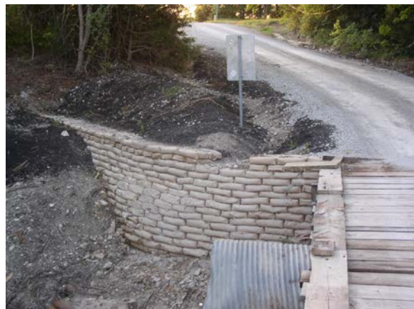
Figure 12 – Bridge abutment stabilization: Stack cement bag bulkhead with ditch outlet
