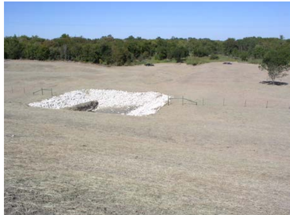
Figure 15 – Floodwater Retarding Structure: Earthfill, shaping and rock lined plunge basin.
