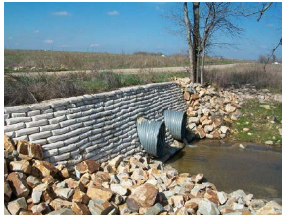
Figure 6 – Road Crossing: Stacked cement bag abutment with rock armor.
