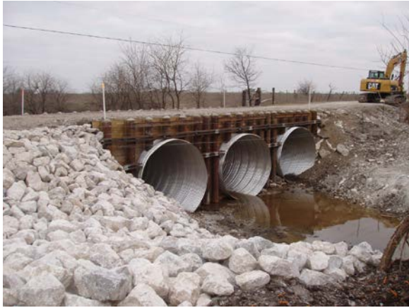
Figure 7 – Road Crossing: Timber abutment with rock chute
