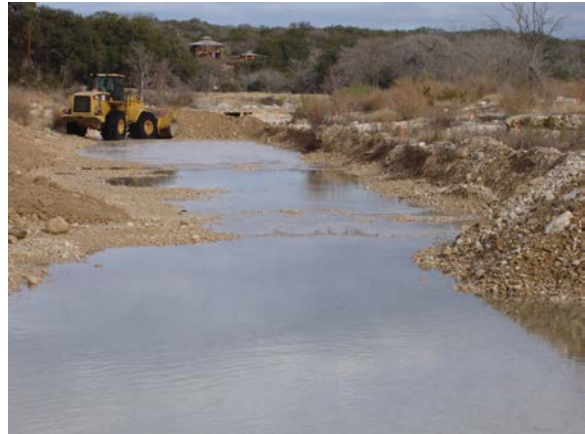
Figure 14 – Silt and gravel removal for stream channel
