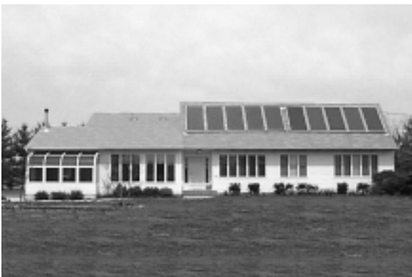
Ten flat-plate solar collectors heat water for this home in Elm, New Jersey; its many south-facing windows reduce heating bills in winter.
