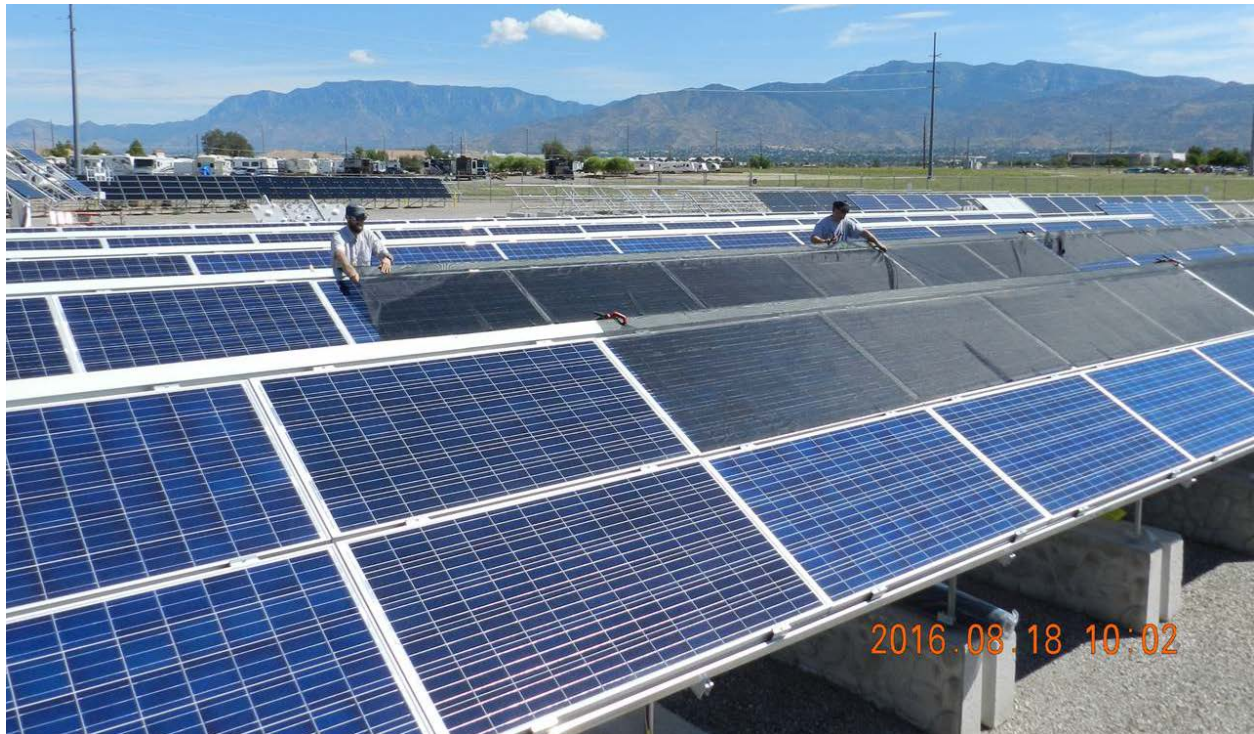
Figure D.1. Shading mesh applied to both rows of the Maxim installation.
