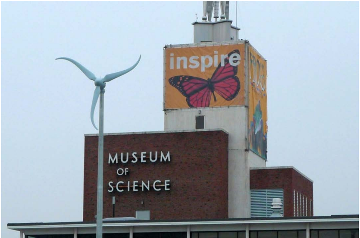
Figure 10. Skystream installation at the Boston Museum of Science. Photo from Boston Museum of Science, NREL 18006
