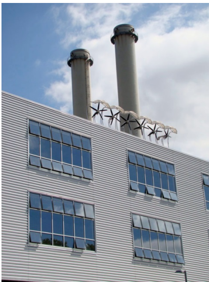
Figure 11. Brooklyn Navy Yard wind turbine installation. Photo from Flickr 2874788682
