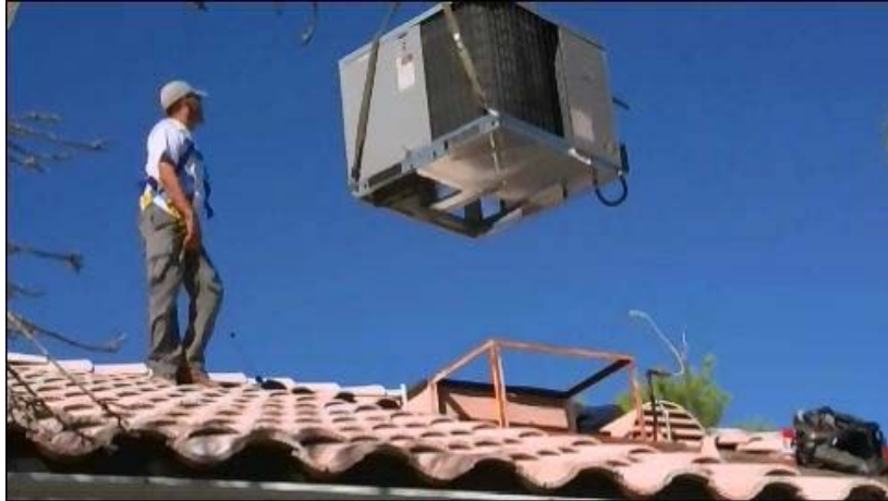
Figure 9. Old equipment removal from Las Vegas community-scale retrofit project
