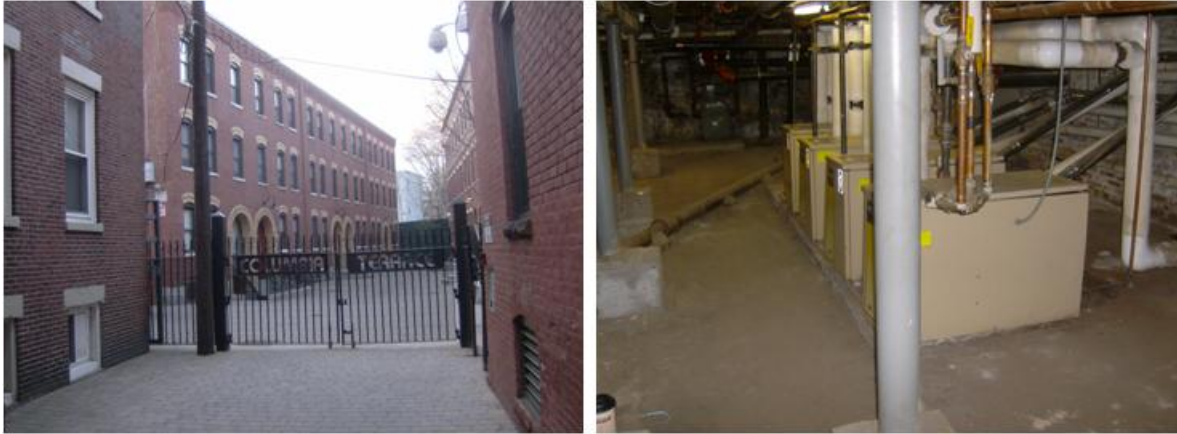
Figure 7. Exterior view of test building and typical basement boiler room
