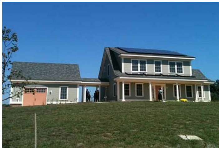
Figure 11. The National Institute of Standards and Technology Zero-Energy Test Facility
