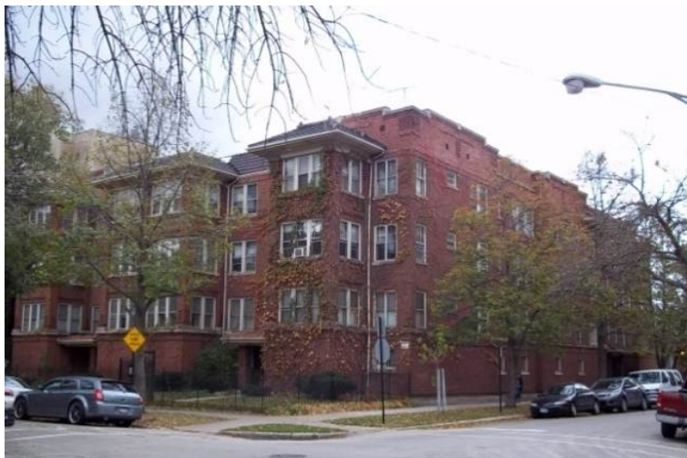
Figure 16. A typical building that could benefit from steam system balancing and tuning
