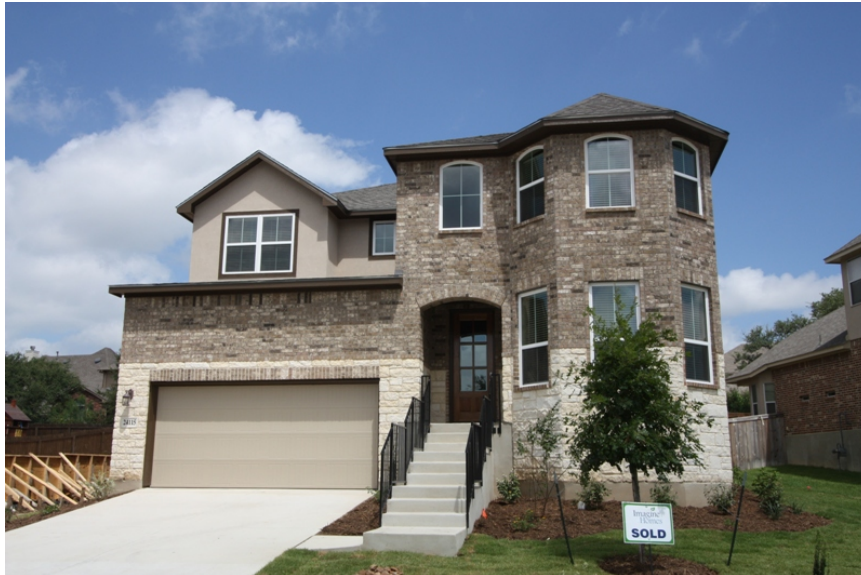
Figure 13. Imagine Homes test house in San Antonio, Texas
