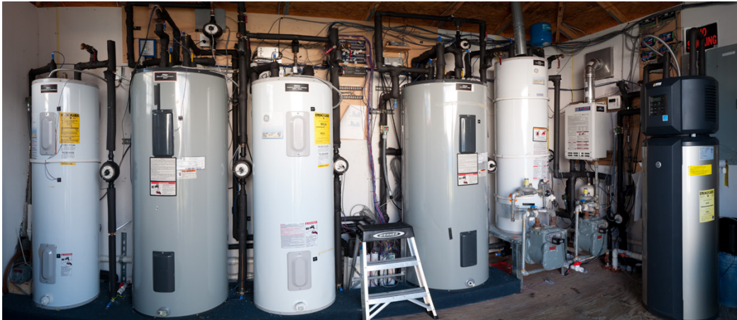
Figure 10. The FSEC water heating laboratory
