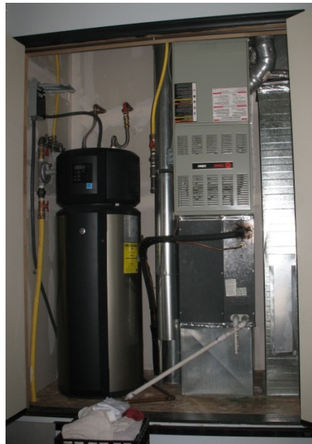
Figure 13. GE GeoSpring HPWH installed in garage closet
