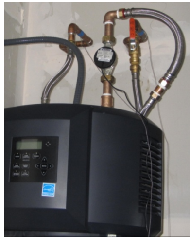
Figure 17. Final plumbing configuration with the flow meter and an extra length of flexible pipe installed
