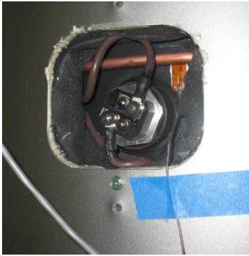
Figure 2. Surface-mounted TC is secured while the epoxy cures.
