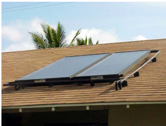
Figure 2. Flat-plate collector
