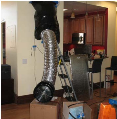
Mini-split heat pump under test. Photo by Xia Fang, NREL/PIX 18336
