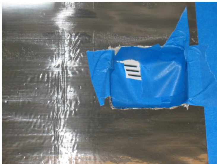
Figure 27. Opening for unit room temperature thermistor sensing
