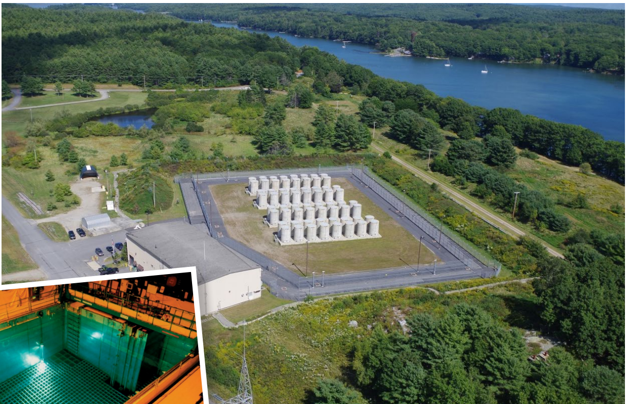
Independent spent fuel storage installation at Maine Yankee site.
