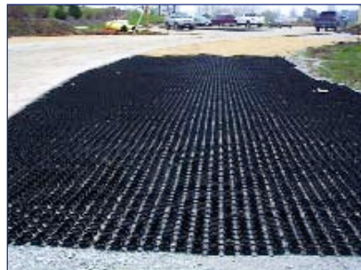
Sub-structure of grass paving.
