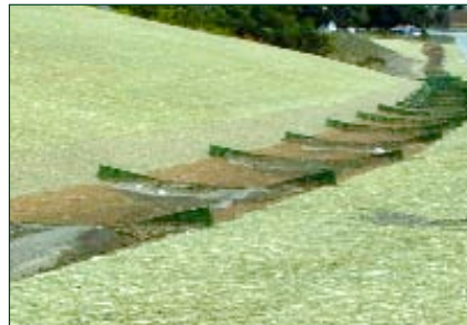
A GeoRidge™ system complements erosion control blankets to protect areas of concentrated flow on this site in Iowa's fragile Loess Hills region.
