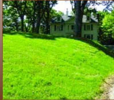
Compost blankets control erosion until seeding is adequately established.
