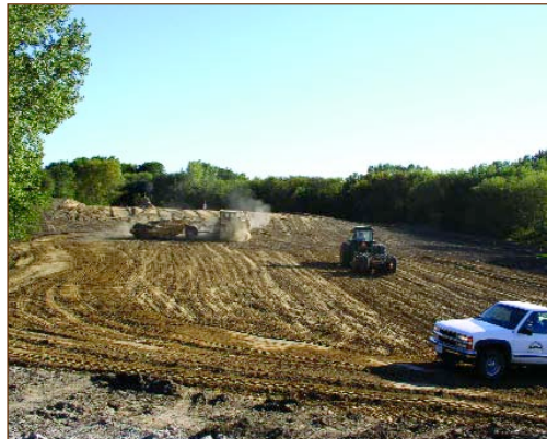
Minimize the amount of land exposed to erosive rain and wind with phased grading.
