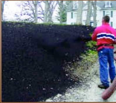
Applying compost and seed with a pneumatic blower truck.
