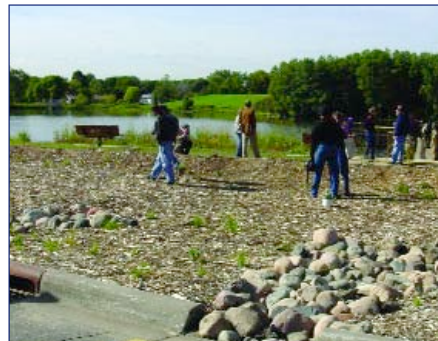
A turf island was converted into a bioretention cell at this site. Curb cuts allow runoff to enter the bio-cell for pollutant removal. Large runoff events can still enter storm sewers.
