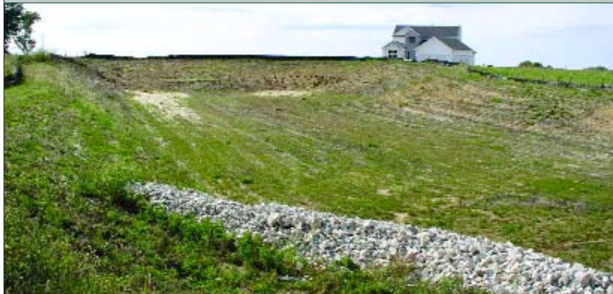
The rock check dam shown above adds water quality protection to a traditional storm water detention basin by temporarily impounding runoff from frequent, low intensity rainfalls. A traditional detention basin only controls large storms to reduce flooding.
