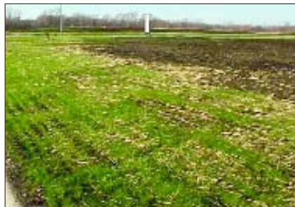
Straw mulch was disked in where vegetative cover is starting to establish. The mulch blew off the bare ground to the right because it was not tacked in by disking.
