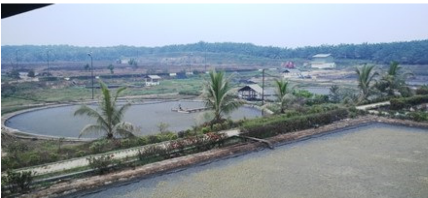
Palm oil mill effluent (POME) ponds at the PT Nirmala Agro Lestari mill in Lamandau District. DOE's SERIG project developed technical and economic analysis for generating renewable electricity from the biogas emitted from the effluent ponds at this and another nearby mill. This would provide power for the mills and nearby communities.
