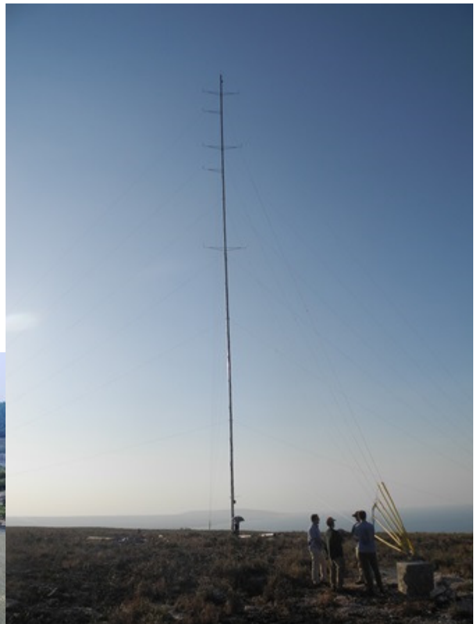
A 60-meter meteorological (met) tower was installed on Sumba Island by Winrock International (contractor to DOE's National Renewable Energy Laboratory on the SERIG project) to collect data on the quality of the site's wind resource in preparation for development of a wind project (funded by the Asian Development Bank).
