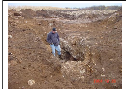
Sinkholes can be stabilized to minimize erosion and groundwater contamination. Photo by DCSWCD
