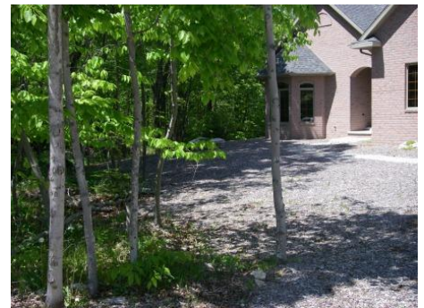
Building pads that filter storm water blend into the landscape after construction, as green space or heavy mulch cover. Photo by DCSWCD
