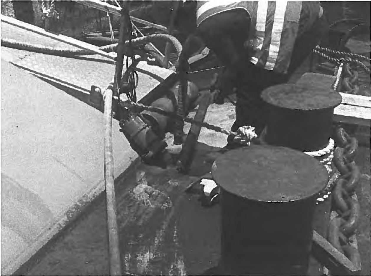
Sump and hose used to remove stormwater from deck of drydock.
