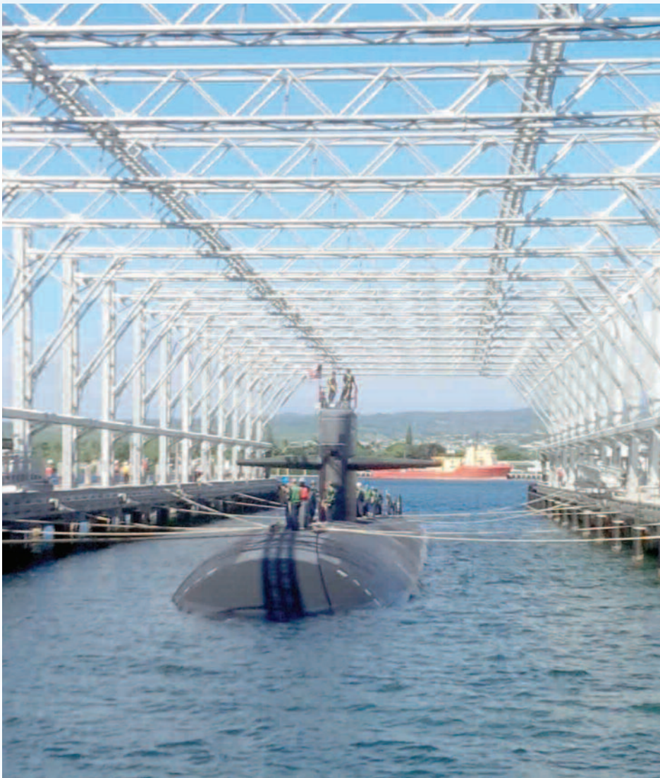
(Above) The Pearl Harbor magnetic silencing facility (MSF) team completed a successful magnetic treatment (deperm) event Nov. 25. Joint Base Pearl Harbor-Hickam has the only drive-in submarine deperm facility in the Pacific Fleet area of responsibility (with two certified deperm engineers) and a state-of-the-art type 6 electromagnetic measurement range. This enables the U.S. Pacific Fleet submarine force to maintain its magnetic stealth capability.
