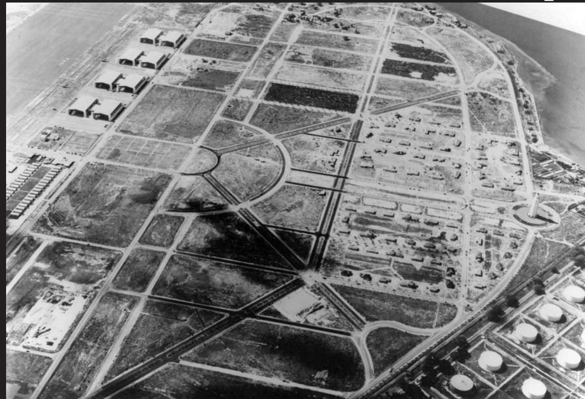
Photo courtesy of the Hawaii Department of Transportation Aviation Division
