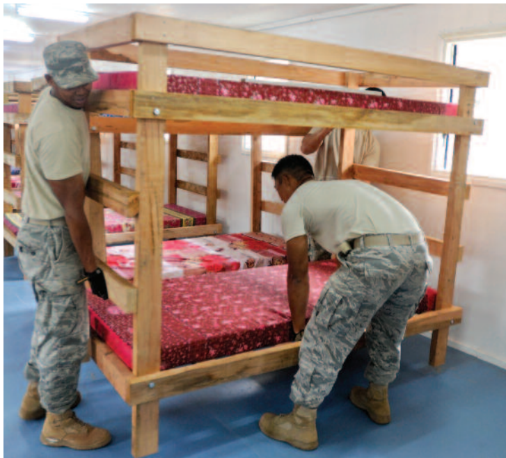
Members of the Hawaii Air National Guard 154th Civil Engineer Squadron move bunk beds into place inside a newly built dormitory at Togoba Secondary School as Pacific Unity 14-8 in Mount Hagen, Papua New Guinea wraps up.
