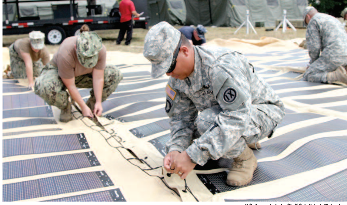
U.S. Army photo by Staff Sgt. Kyle J. Richardson Sgt. Roy Gano, a carpenter/masonry technician with the 871st Engineer Company, 9th Mission Support Command, along with other support elements, becket-lace the solar shade canopy together during the setup of a humanitarian aid and disaster relief event for Rim of the Pacific 2014 training exercise at Ford Island on July 7.
