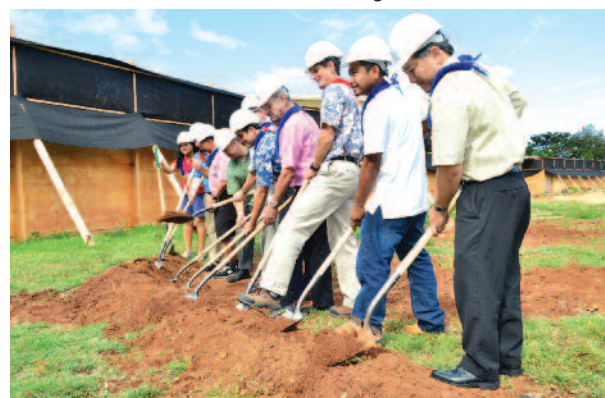
Hickam Elementary faculty members, JBPBH personnel and Hawaii State Rep. Aaron Ling Johanson celebrate the construction of a new library at the school with a groundbreaking ceremony held June 17 at Hickam Elementary School.
