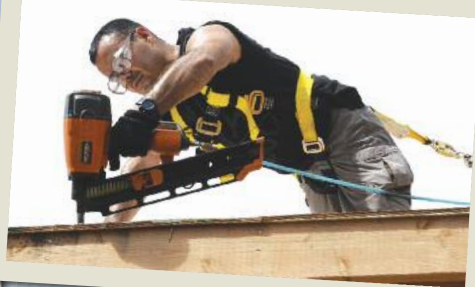
Tech. Sgt. Manny Garibay, 15th Maintenance Group, uses a nail gun to secure plywood on a rooftop.
