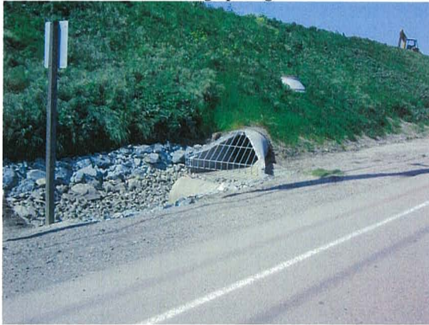
Photograph 5: Pacific Ethanol storm drain outfall into the drainage channel along Navy Drive.
