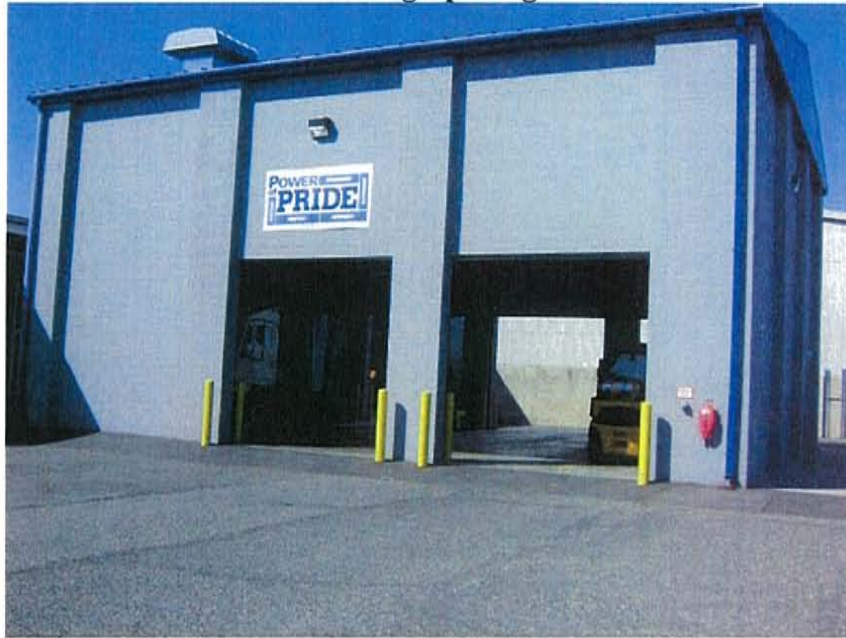
Photograph 11: View of Lowe's Distribution Center equipment maintenance shop.
