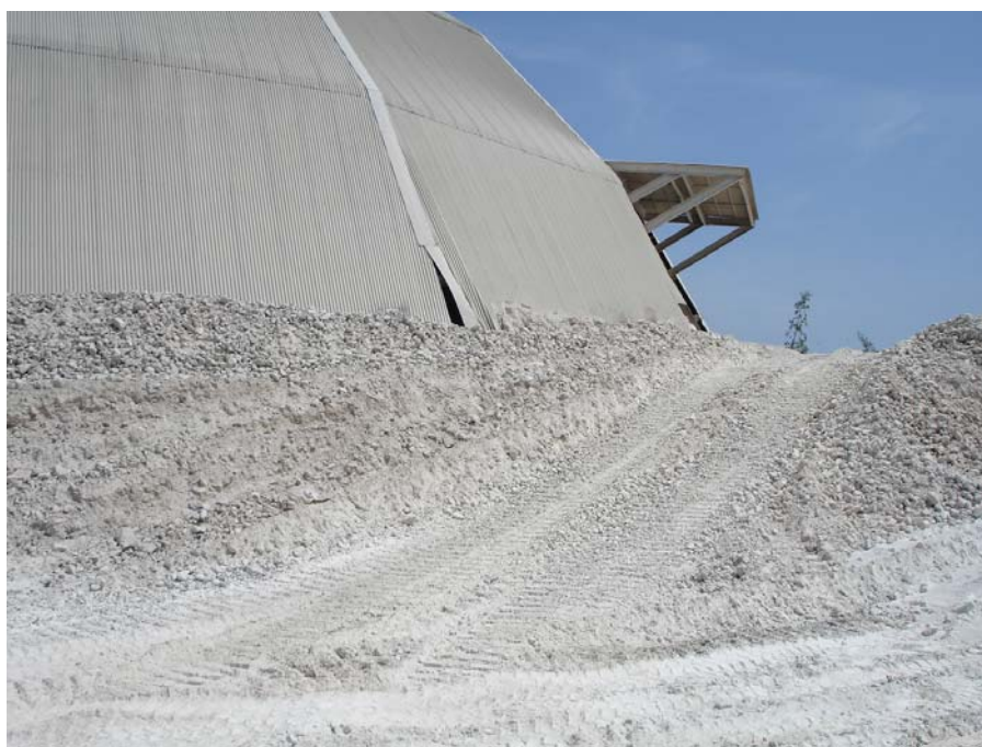
Photo 2: Pile storage of gypsum rock and associated fines. The pile, located on the northwest side of the facility, is partially covered by a dome.
