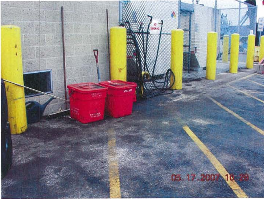
DCN0446 – View of filling area at lube oil station. Note stains, lack of containment at this area.
