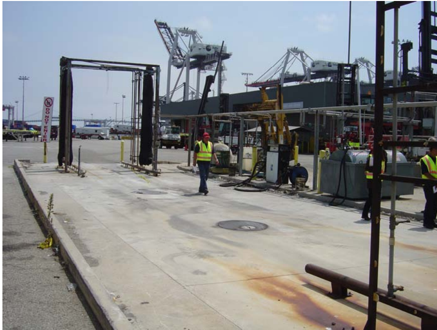
Photo 3: The vehicle and container wash rack area.
