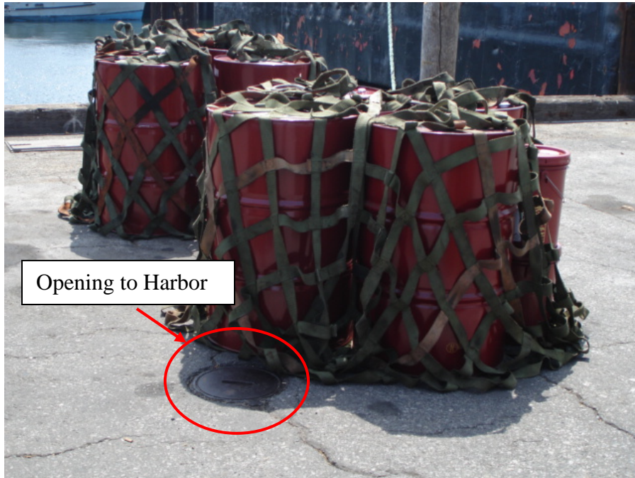
Photo 5: Oil drums at uncontained area adjacent to the wharf, directly next to opening leading to the Harbor.
