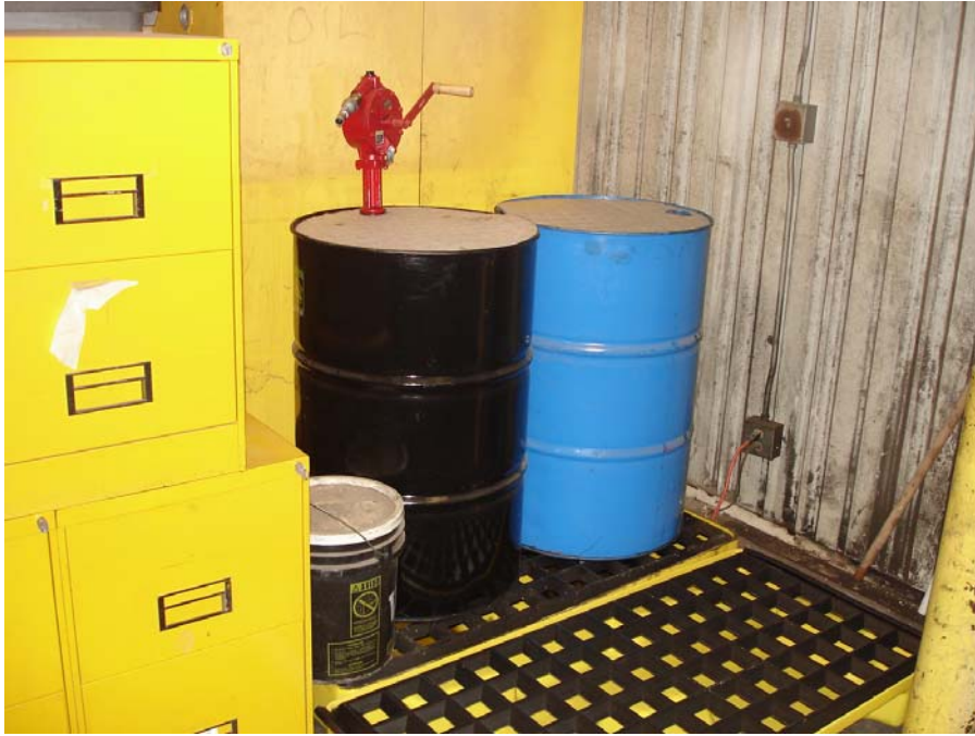
Photo 3: Indoor storage and containment were provided for oil drums.
