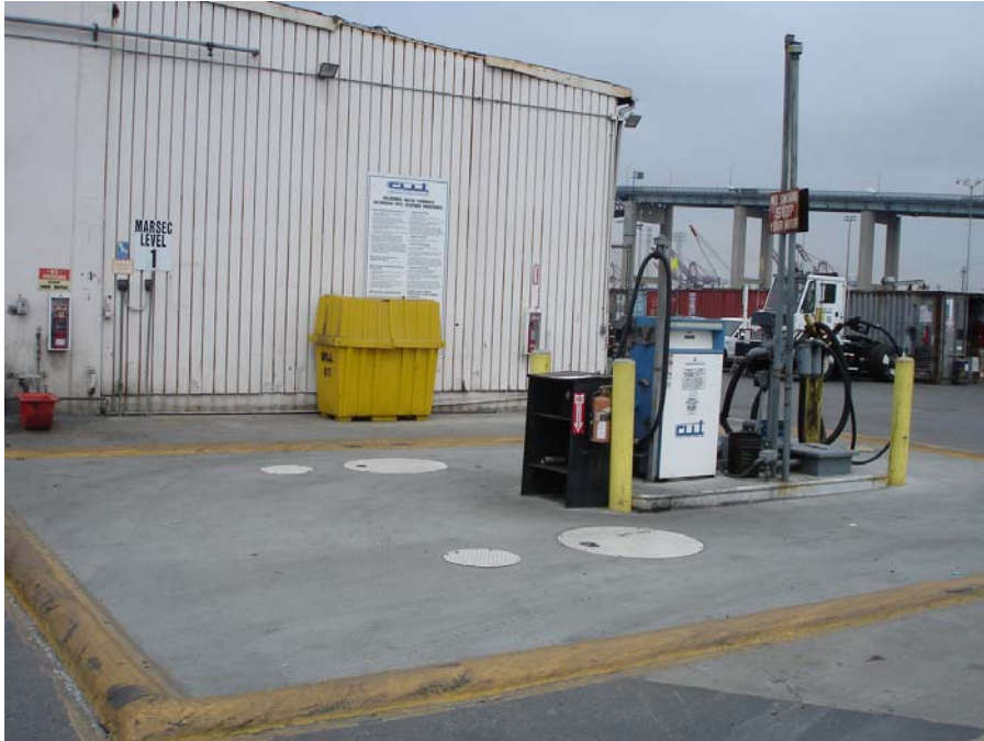
Photo 3: Bermed fueling area at maintenance shop.
