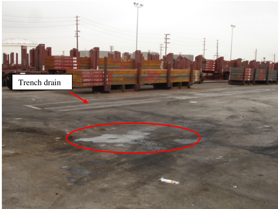
Photo 3: Exposed oil leak near rail yard trench drain.
