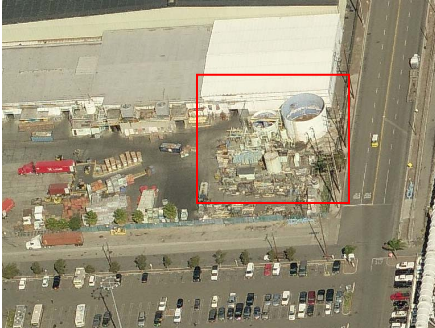
Photo 2: Storm water treatment plant.
