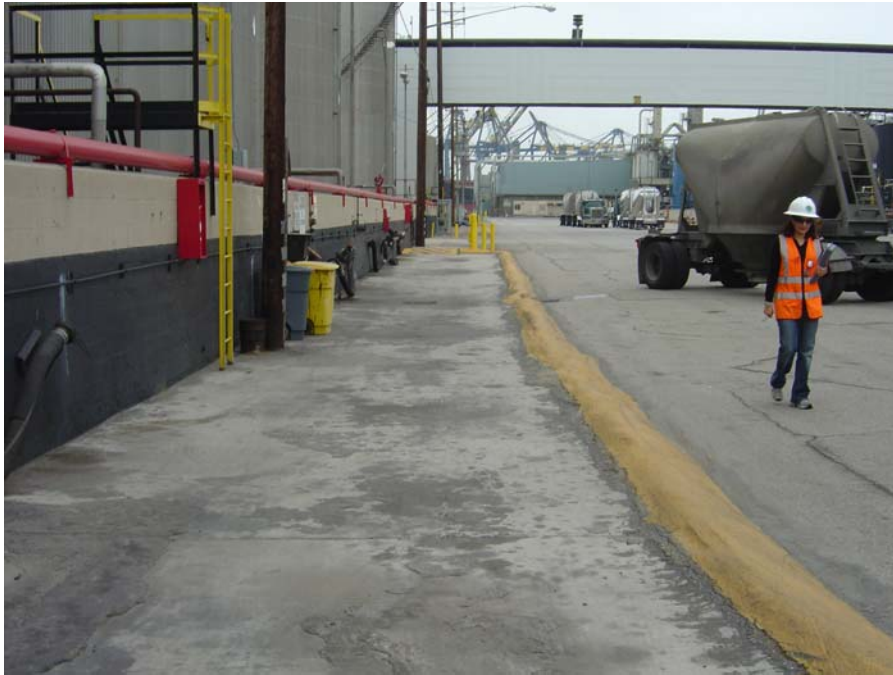
Photo 1: Housekeeping throughout the facility was good (area east of tank blocks shown).
