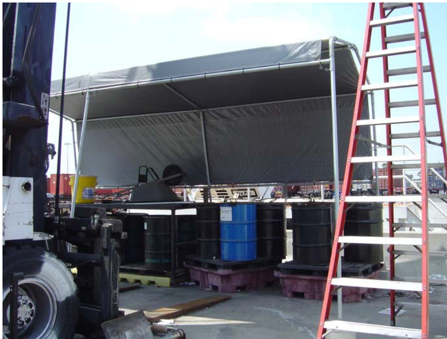
Photo 4: Drum storage area adjacent to the maintenance area. All drums were observed under cover and on spill pallets.
