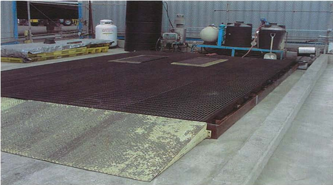
4. Vehicle washing rack within a berm - The washed water is filtered and reused in the same area.
