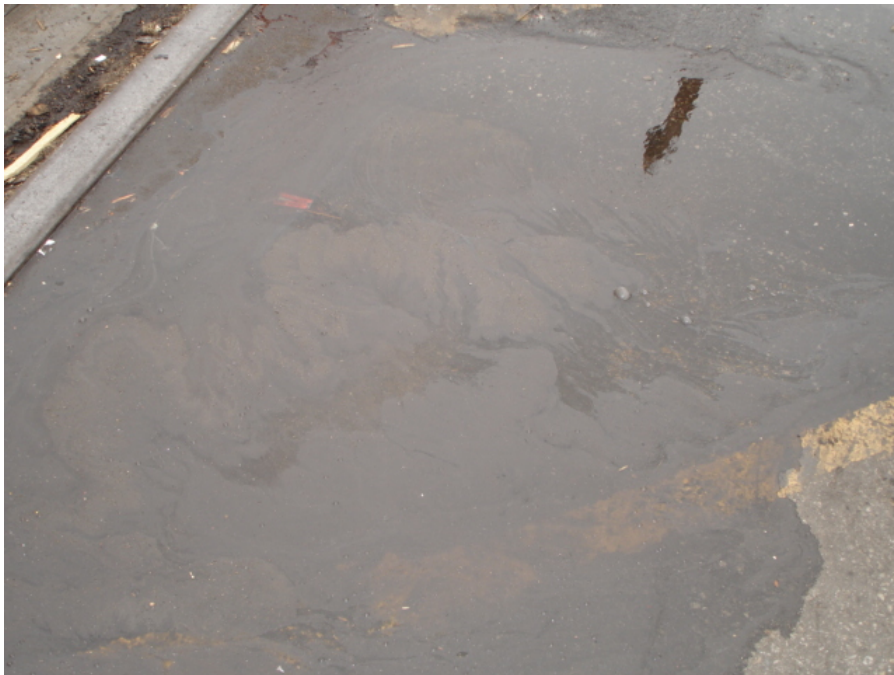
Photo 11: Condition of water leaked from container pictured above.
