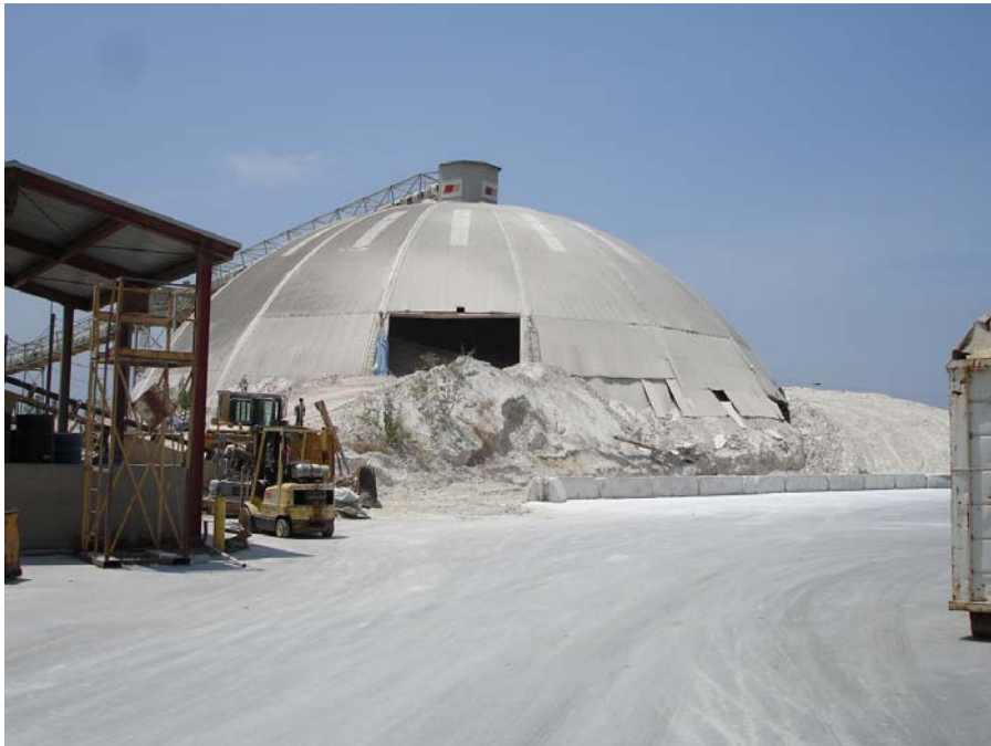
Photo 2: Pile storage of gypsum rock and associated fines. The pile, located at the southern end of the facility, is partially covered by a dome. The covered conveyor leads from the unloading dock.
