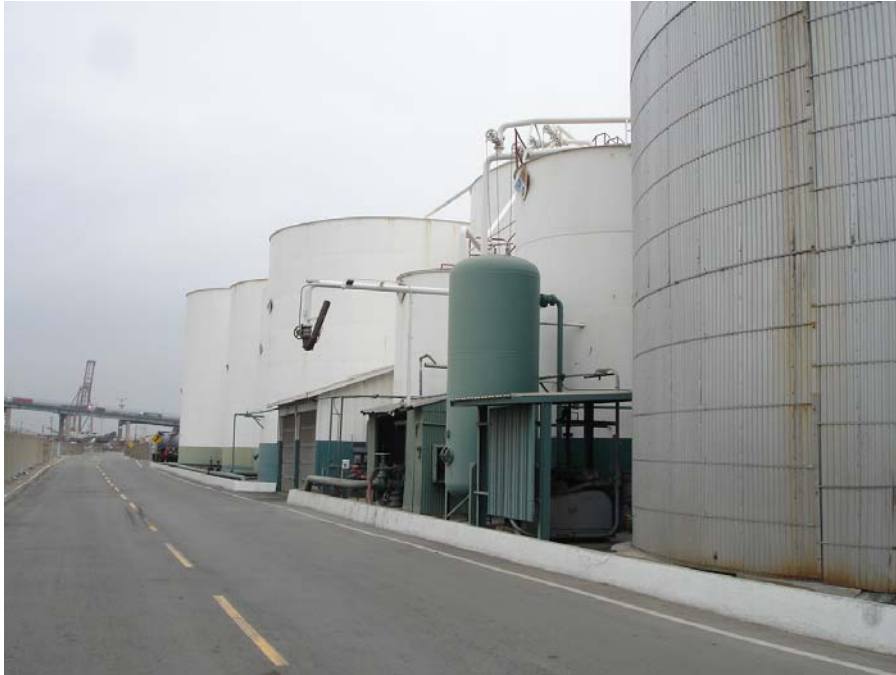
Photo 7: Tank truck rack on west side of the facility.
