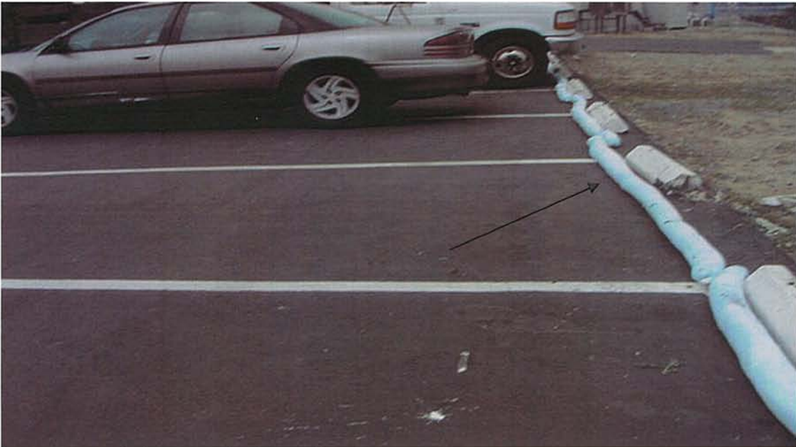
2. Storm wattle is placed in the parking lot area.
