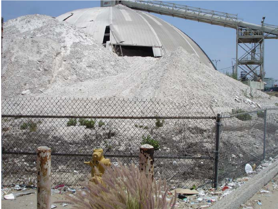
Photo 3: Gypsum pile at southwest corner of the facility. The photo was taken from the location designated as “Outfall 002” on the facility’s site map. From visual observation, it appears this area would receive run-off from the pile of material shown.
