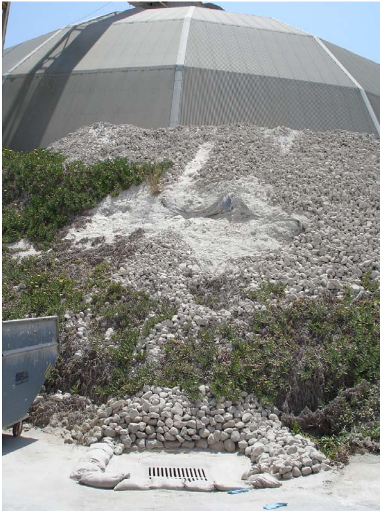
Photo 5: Storm drain directly next to outdoor gypsum storage and associated fines.
