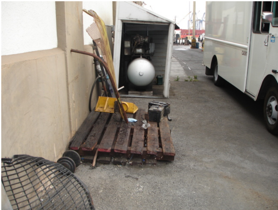
Photo 9: Vehicle batteries at exposed area near maintenance shop.
