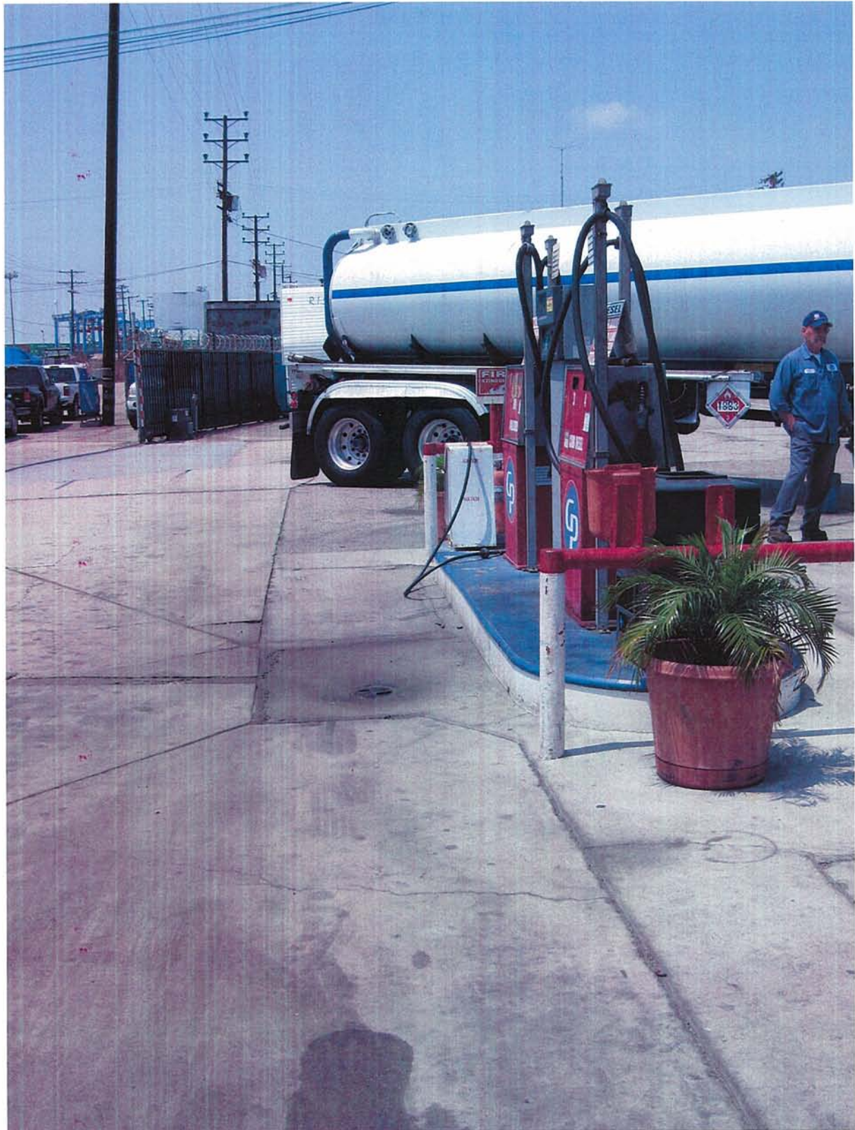
Photo 1: Fueling Area, drain leads to oily water catchbasin
