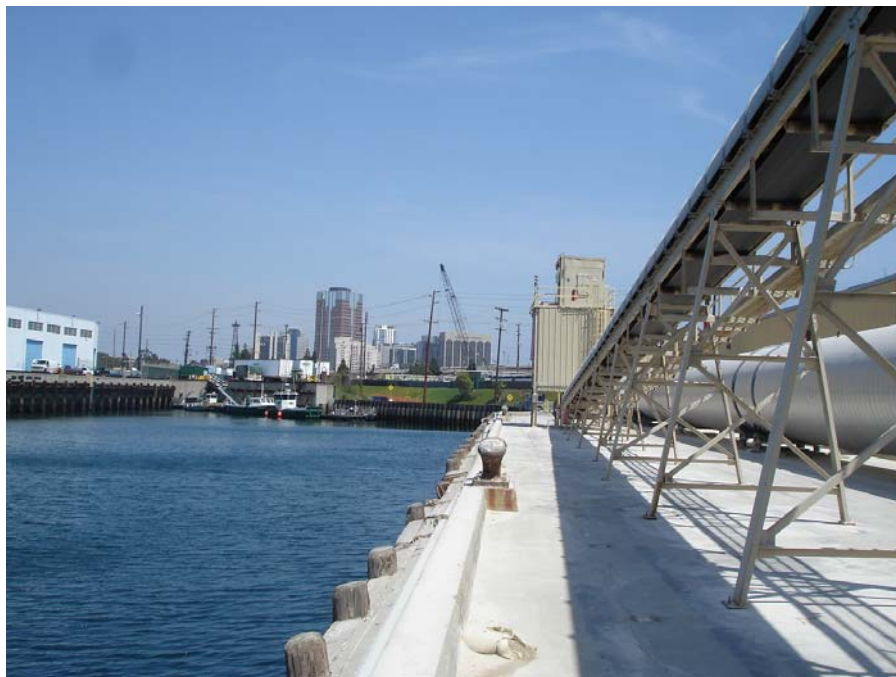
Photo 8: Ship unloading dock and covered conveyor on the north side of the facility.
