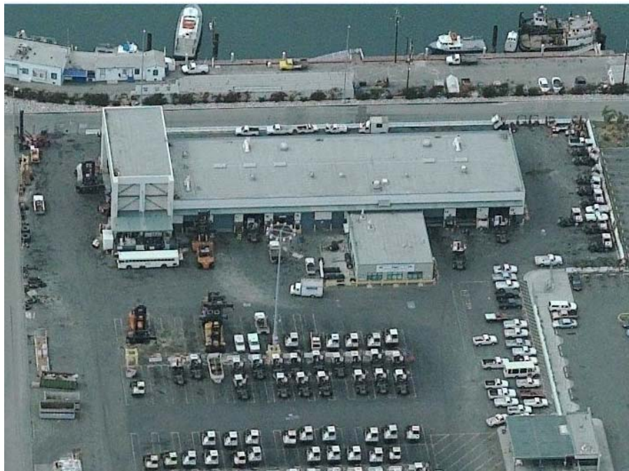
Photo 2: Vehicle maintenance shop (power shop)
