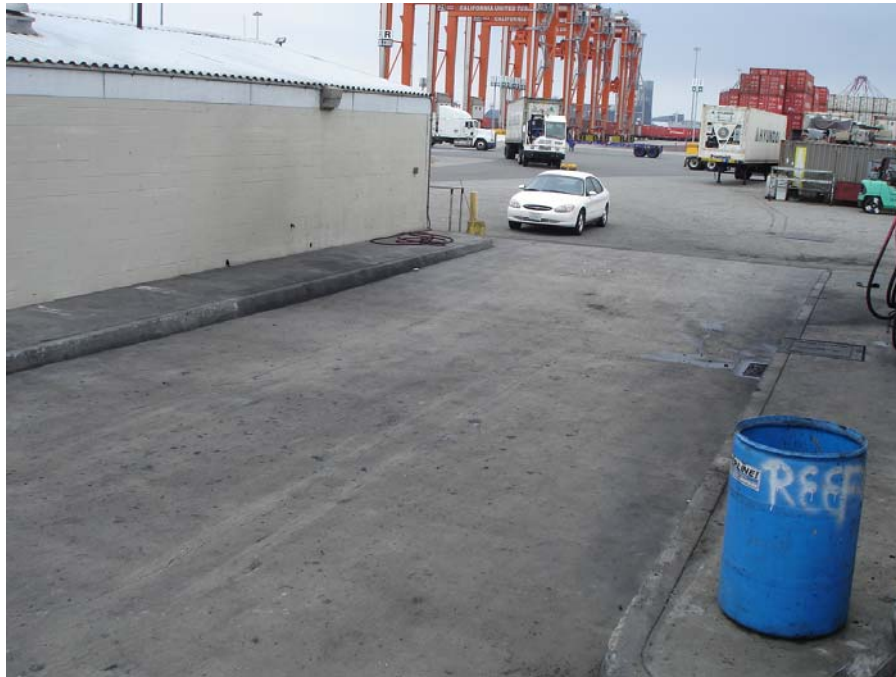
Photo 5: Vehicle wash area directed to sanitary sewer system.
