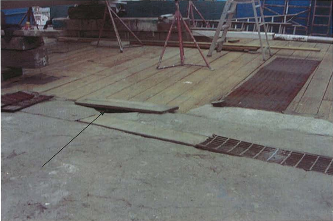
5. Discharge point #1 in the Boat Repair and Dry-Dock Storage area.
