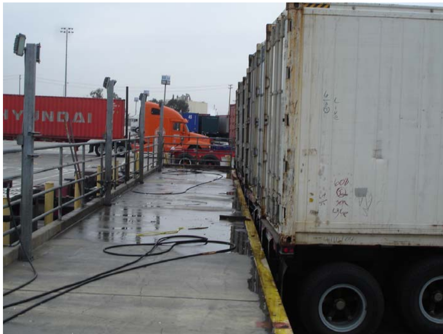
Photo 6: Bermed container wash rack directed to sanitary sewer system.
