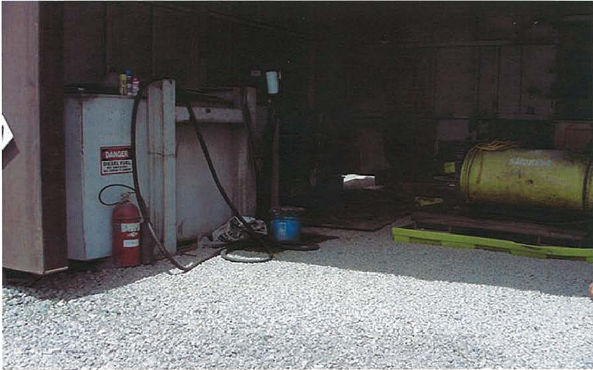
3. Fuels and waste oil tanks are located inside the machine storage shed on gravels.
