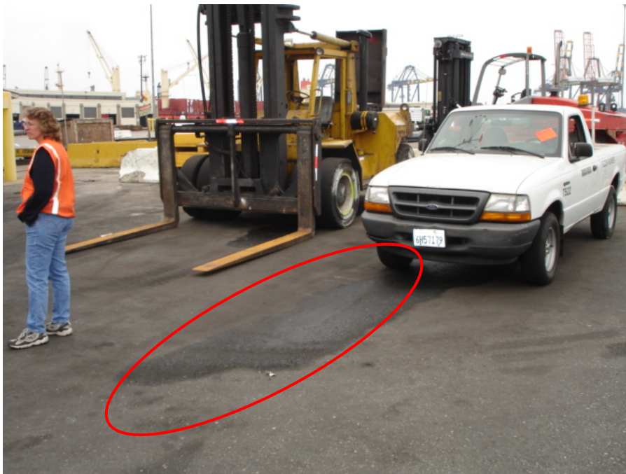
Photo 7: Exposed oil leak adjacent to maintenance shop.
