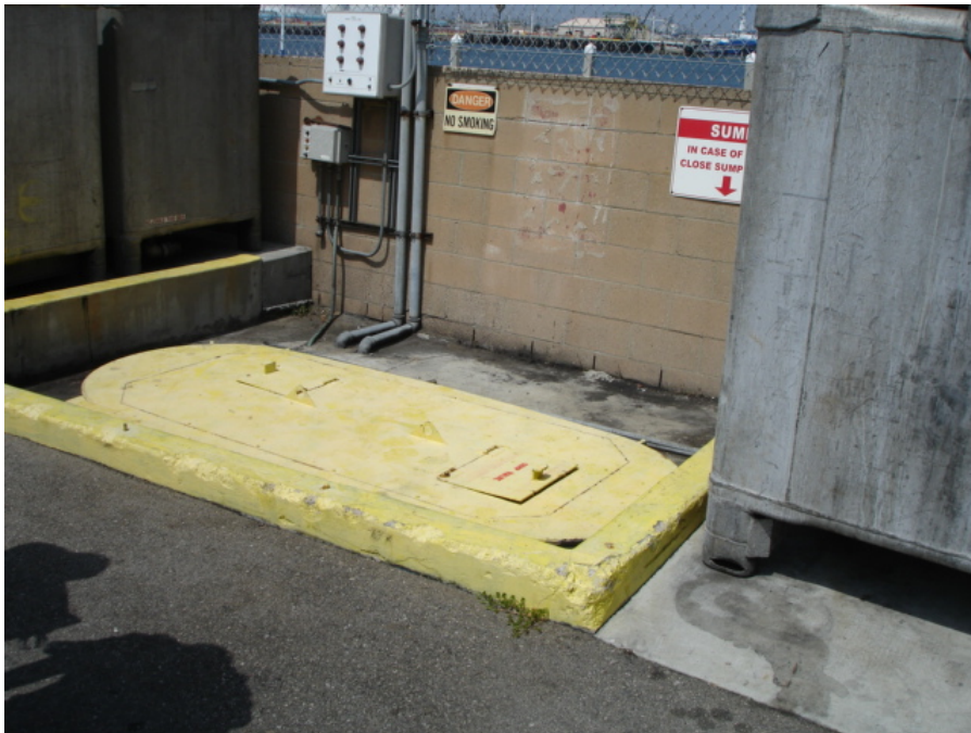
Photo 8: In-ground containment vault.
