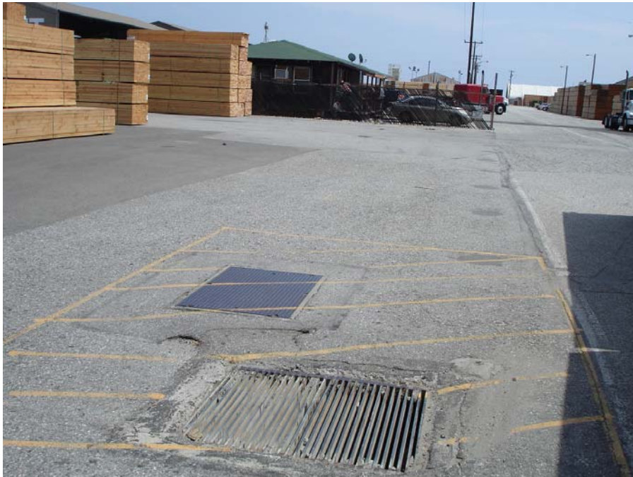
Photo 2: One of three storm drains.
