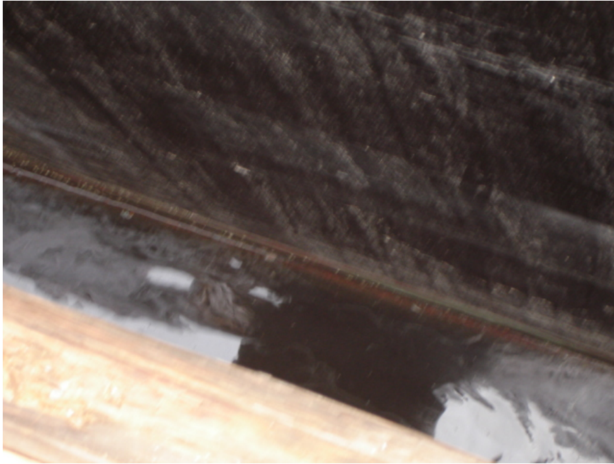
Photo 11: Condition of water between wharf and barge being cleaned.
