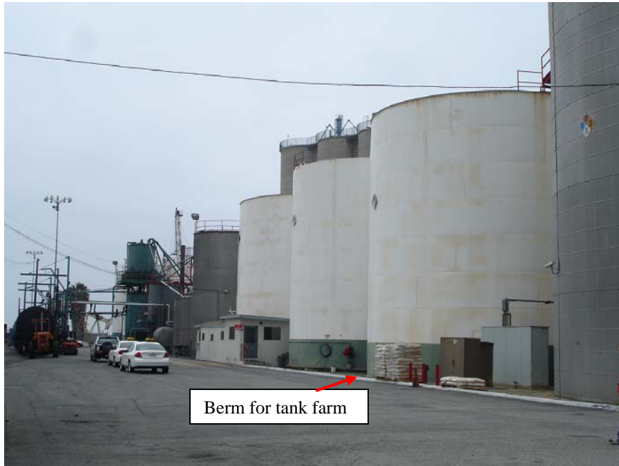
Photo 1: Bermed tank farm.
