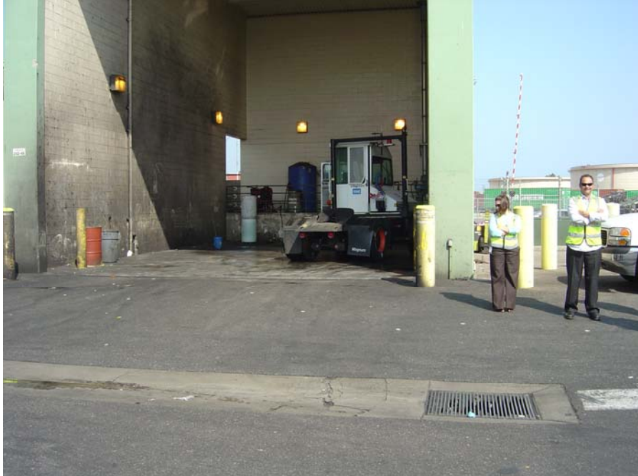
Photo 6: Vehicle/container exterior wash area. Catch basins in this area drain to a oil/water separator for treatment prior to discharge to the industrial sewer.
