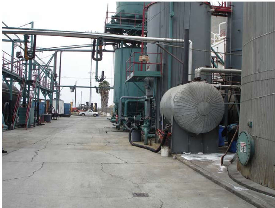
Photo 2: Truck loading rack that drains to sump in tank farm.
