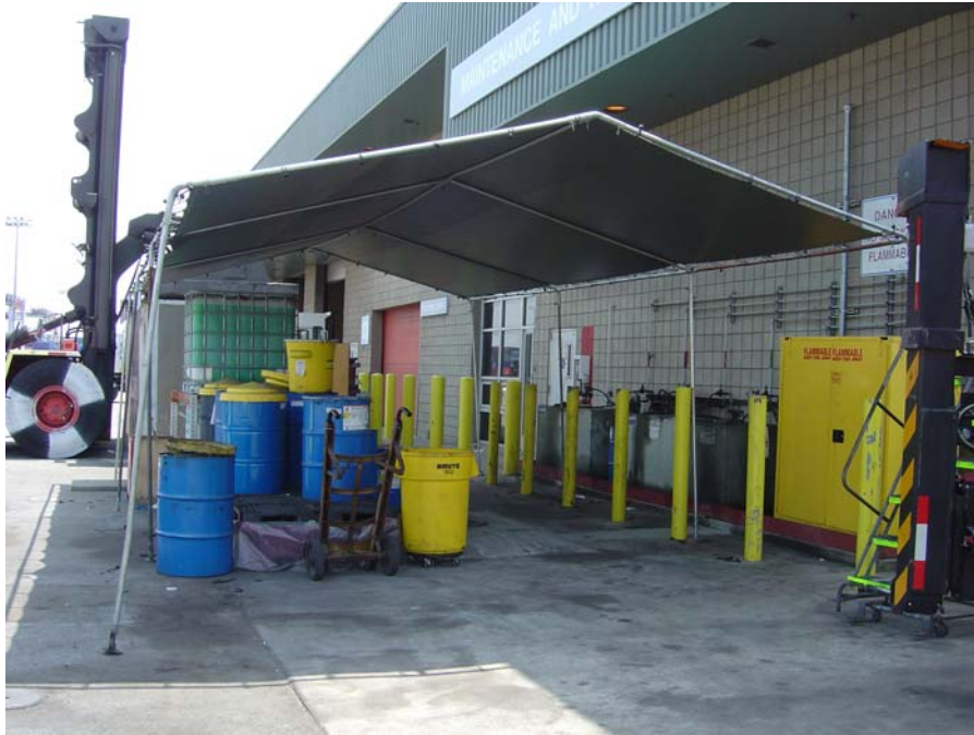
Photo 1: Several drums at the vehicle maintenance area were not on spill pallets.
