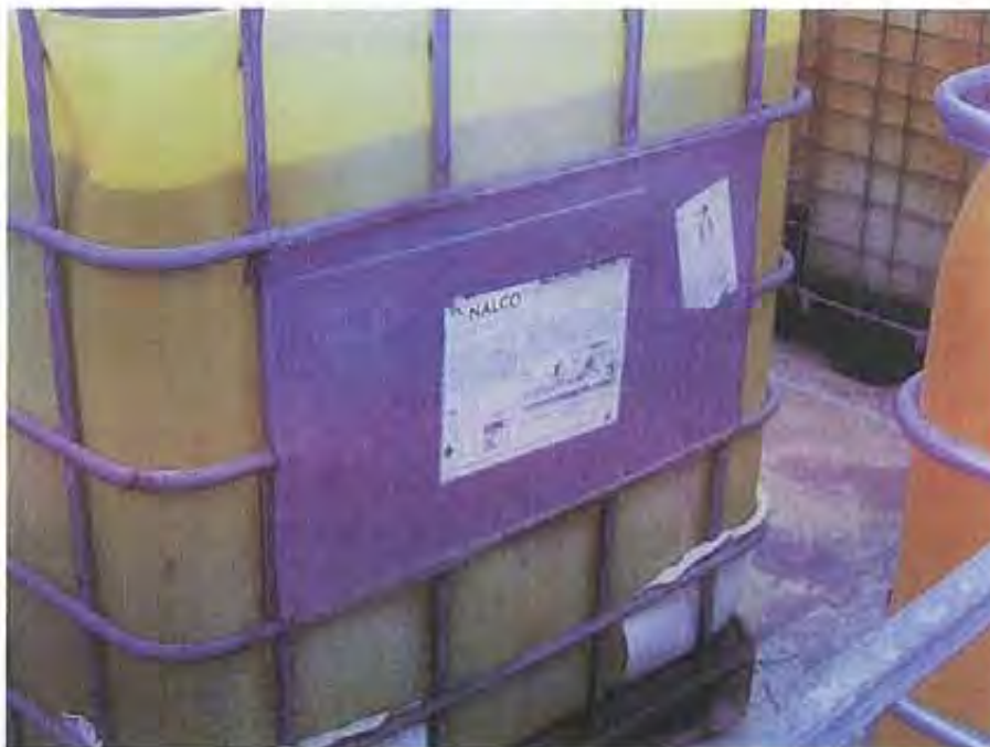
Photo 35: A tote originally used for flocculent was being used to store diesel fuel, without secondary containment. The tote was labeled as flocculent.
