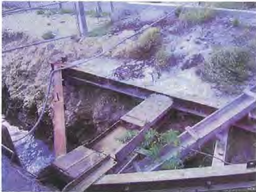
Photo 26: Evidence of concrete spillage from an on-site construction activity (possibly the construction of the concreted area itself or the berm) toward the receiving water. It is unclear if any of the concrete actually entered the receiving water, although concrete observed on the very edge of the metal frame work would indicate that it did. However this photo demonstrates a lack of effective best management practices utilized for the construction project by the Discharger this close to the edge of the receiving water.
