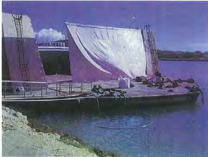
Photo 59: An overview of the Lil' Parris dry dock facing northeast.
