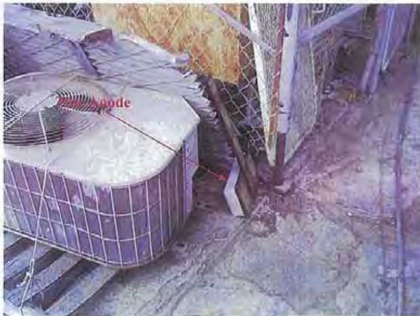
Photo 46: Another zinc anode observed on the deck of the work barge, exposed to potential storm water runoff.
