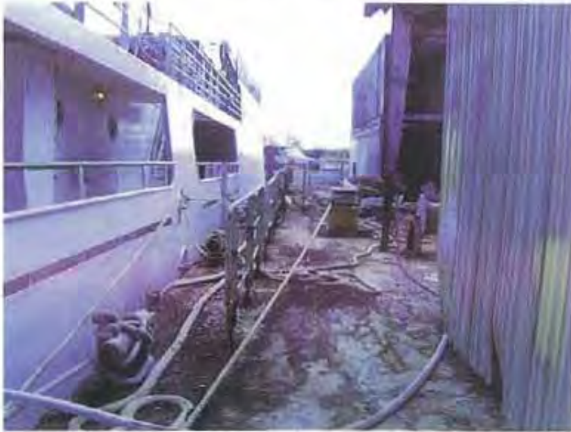
Photo 40: The floor of the work barge was covered in general debris and rust chips/dust, exposed to potential storm water runoff.
