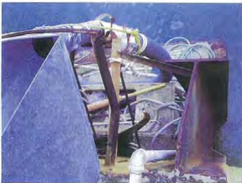
Photo 45: A sink was observed on the stern of the work barge. The Facility representative stated that he believes the sink discharges directly into the harbor below. The Facility representative stated that the sink is used for washing hands and cleaning fish. Due to the location of the sink, it was not possible to confirm the discharge location of the sink.
