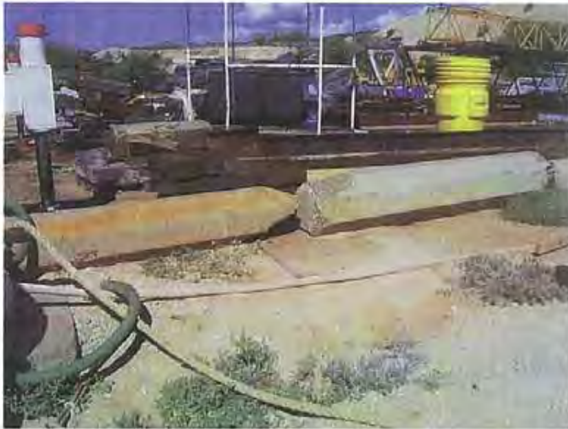
Photo 48: The shore side staging area for the Lil' Perris dry dock has a berm built from cement pillars. Plastic sheeting has been laid down against the pillars and covered with dirt, however the plastic sheeting has torn away in most areas and gaps are prevalent along the entire berm.
