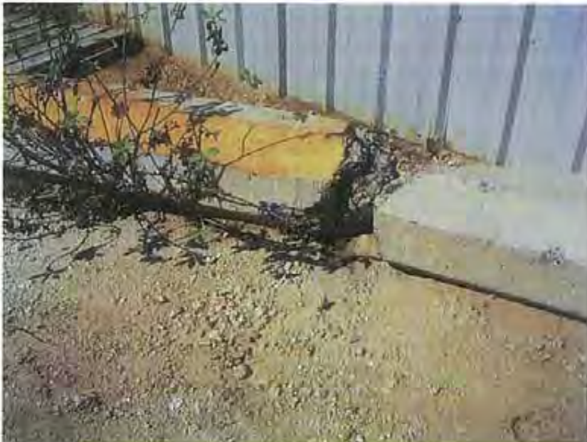
Photo 49: One of the gaps in the berm surrounding the shore side staging area for the Lil' Perris dry dock.
