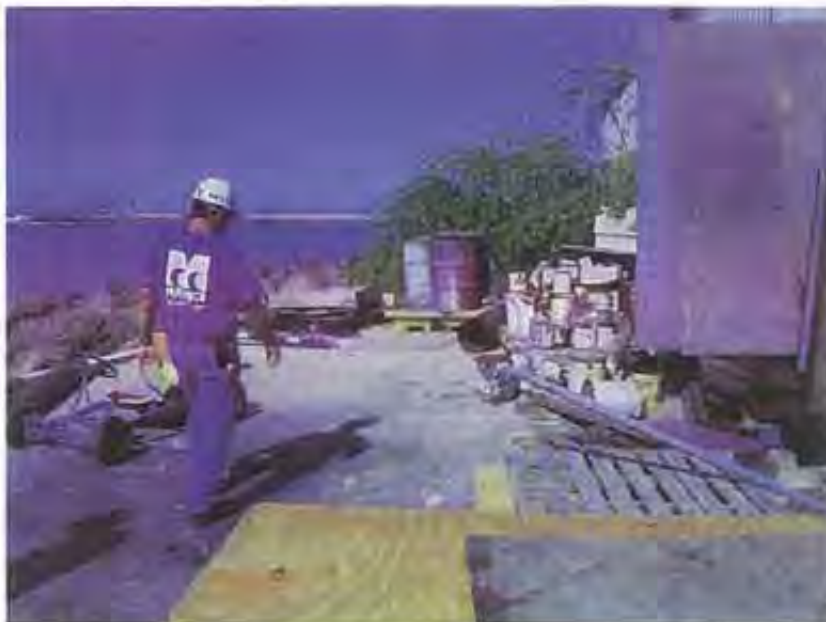
Photo 19: An area northwest of the main yard, behind the metal working building appears to be used for material storage. Materials stored in this area include paint, zinc anodes, and 55-gallon drums. This area does have a containment berm, which directs all storm water to a storm water discharge location pictured in Photo Nos. 23 and 24. A pallet of paint cans was observed stored on-site, exposed to potential rainfall, and in the direct drainage area to a storm water outfall.
