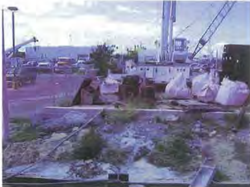
Photo 25: A view from the on-site working barge of the storage area at the southeast end of the main yard. This area was referred to by the Facility representative as "JR's Area". This area has a berm, with identified discharge locations (at the south end of the berm or left side of the photograph, and a gap in the berm to the right where the photograph cuts off). Materials observed stored in this location include used sand blasting grit, heavy equipment, petroleum products, and paint waste (what appeared to be a mixture of paint and paint thinner).
