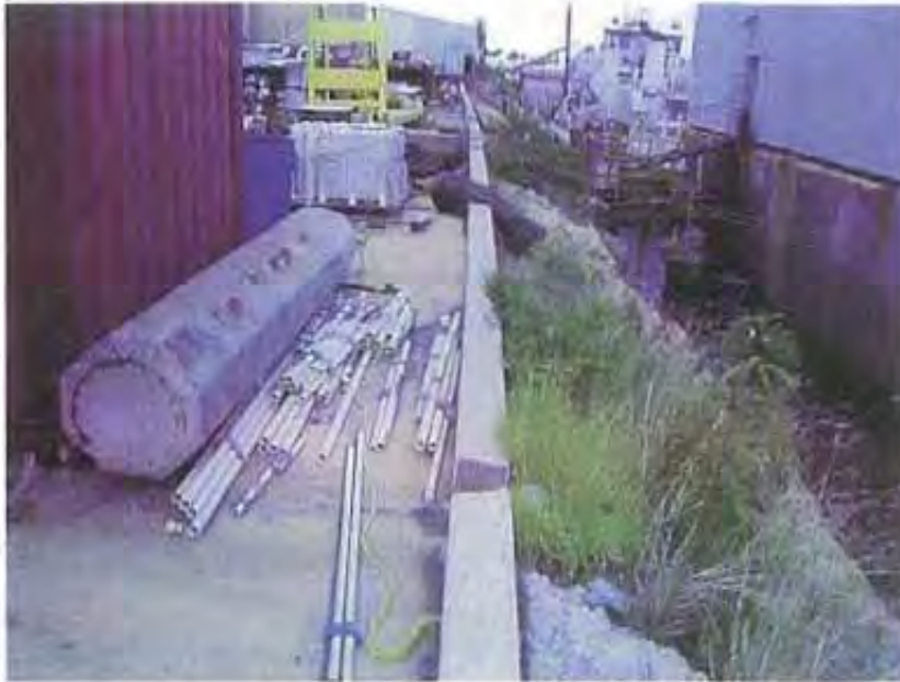
Photo 27: A gap in the berm surrounding JR's area. Discharges through this gap would flow down the bank and directly into the receiving water.
