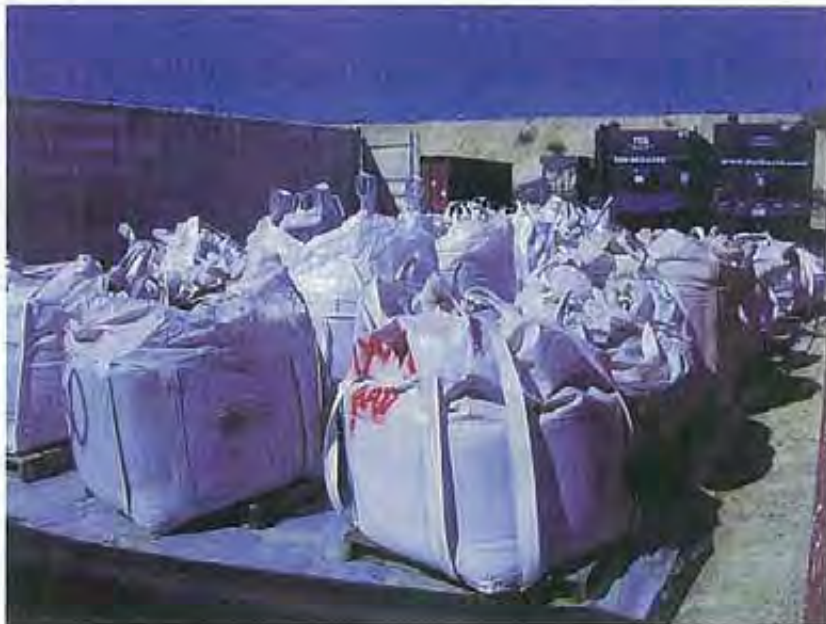
Photo 57: Sandblast grit stored on-site, un-covered.
