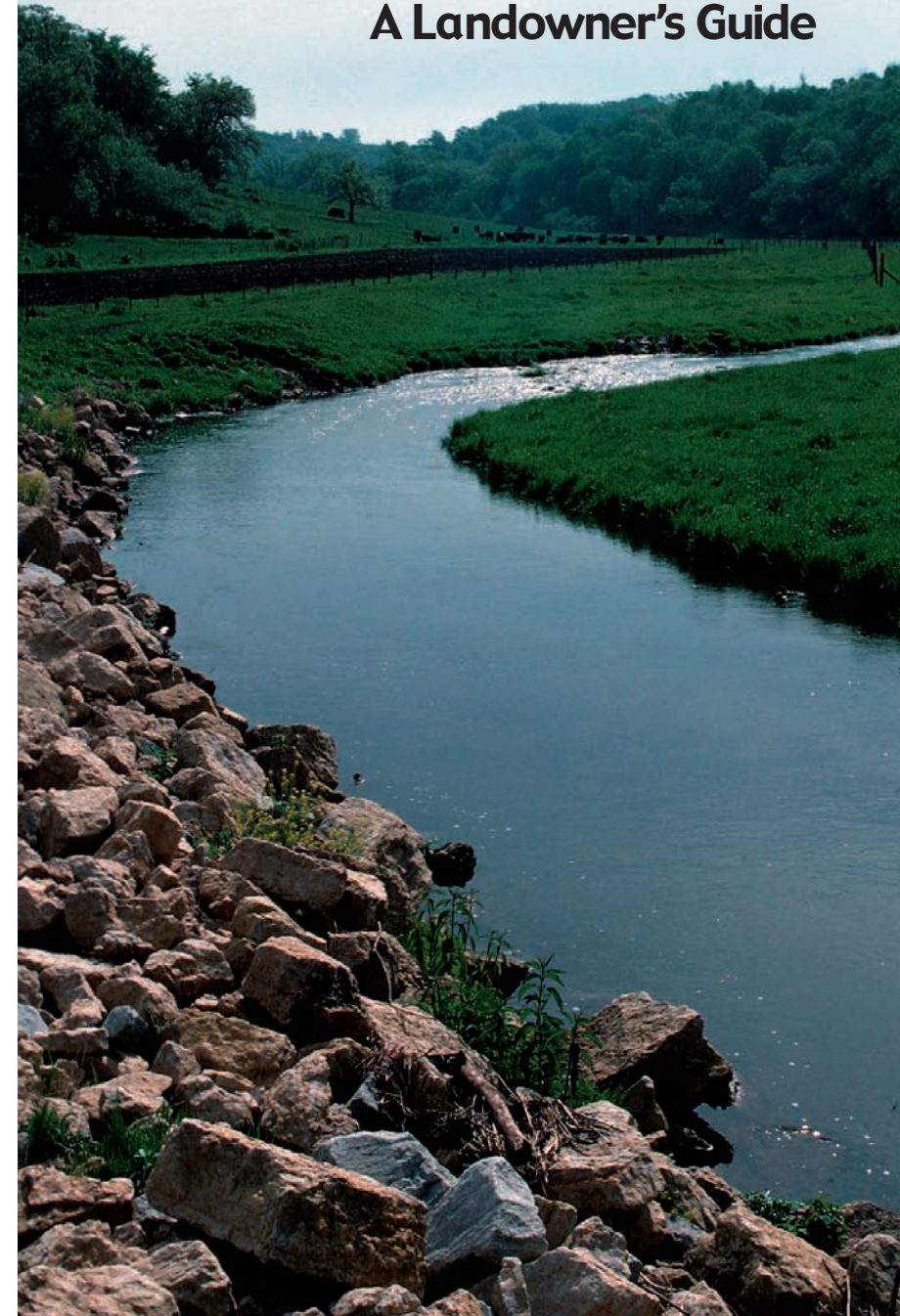
Rip rap is needed to stabilize this streambank to protect the bridge. Many bridges in Iowa are threatened because of channel straightening.
