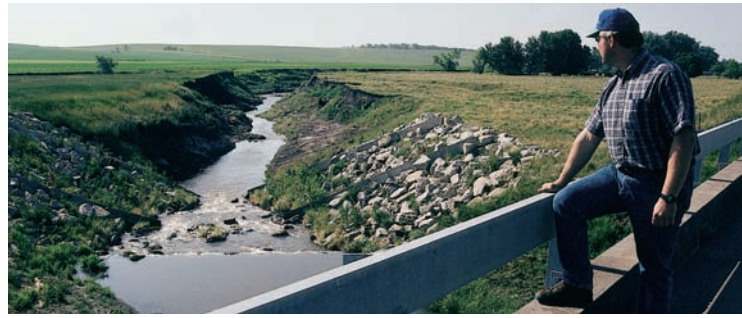
Rip rap is needed to stabilize this streambank to protect the bridge. Many bridges in Iowa are threatened because of channel straightening.
