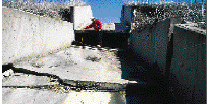
THE PROBLEMS. Dams filling with sediment (top) and deteriorating concrete spillways (above and left) are major, costly problems in the Little Beaver Subwatershed. Dozens of other dams face the same problems.
