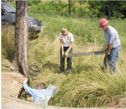
Installing a cave gate
