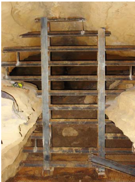
A completed cave gate structure
