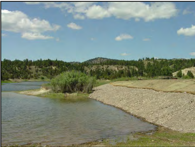
Figure 6. Examples of riprap at Canyon Ferry Reservoir.
