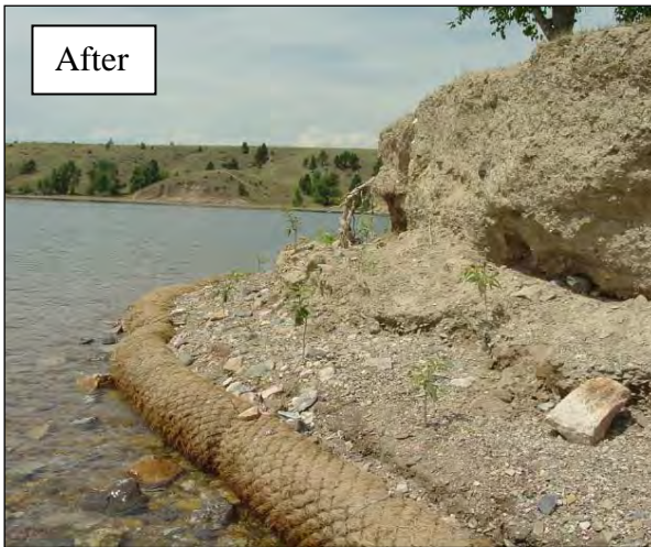
Figure 3. Cave Point is a site where Reclamation has implemented and is monitoring shoreline stabilization measures, including a coir log and cottonwood/willow plantings.
