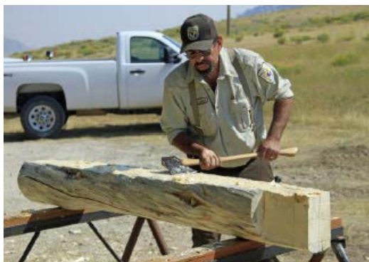
Figure 3: Fernando Escobedo hews the flat side of a log to fit against the backside of the wall's interior paneling.
