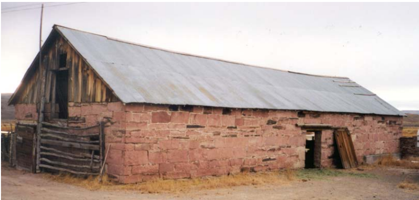
Figure 12. The barn and many other of the ranch buildings are constructed from the distinctive local pink sandstone, some of the blocks weigh up to 300 lbs..
