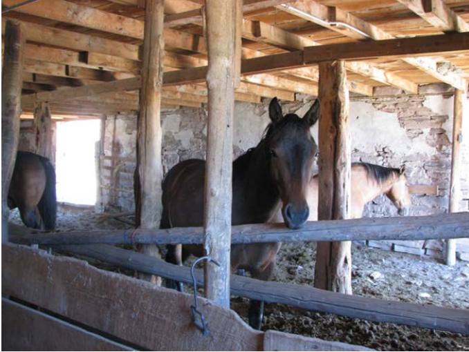
Figure 13. Historically, a horse barn, work recently completed by NPS and Service staff returned that functionality and made the barn available for long-term use by the Refuge.
