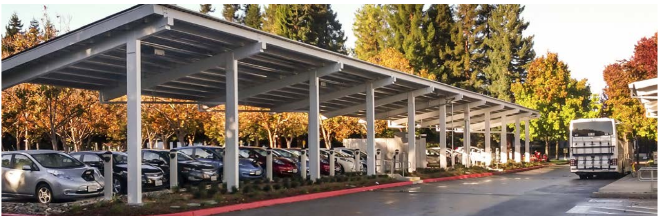
Google is aiming to provide charging at 5% of its parking spaces; it has already deployed more than 300 stations across the country. Photo from Rob Kalmbach, Google, NREL 26459
