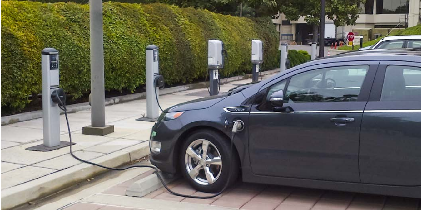
Photo from Southern California Edison, NREL 26481
