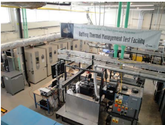
Thermal Test Facility laboratory after construction and equipment installation; Photo credit: Ahmad Pesaran, NREL
