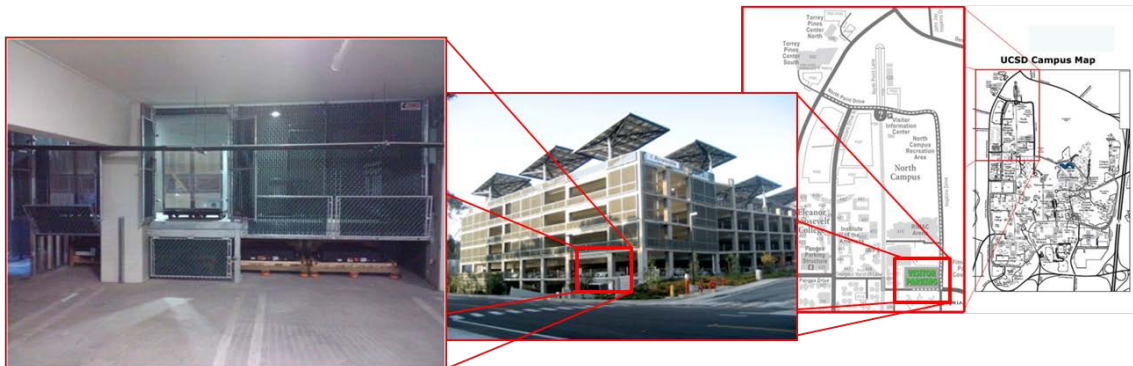
Figure III.C.1.3-4: Second Use Battery Field Test Installation at University of California, San Diego; Photo credits: Jeremy Neubauer, NREL
