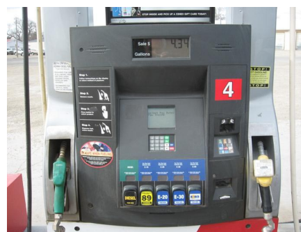
Example of Station Offering Higher Ethanol Blends from the same Hose as E10 (Alleman, NREL)
