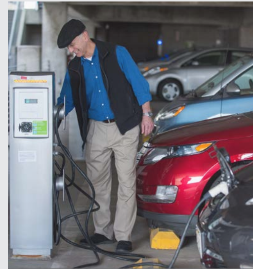
NREL employee Phil Pienkos charges his hybrid vehicle on one of the 36 electric vehicle charging stations in the NREL parking garage.
