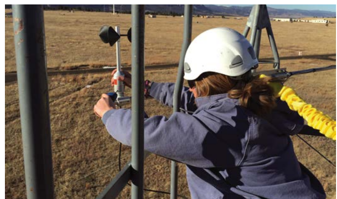
An NREL technician replaces an anemometer on a NWTC meteorological tower. Anemometers provide wind speed data that, along with other data collected, allow NREL staff and industry partners to evaluate the performance of wind turbines under varying environmental conditions. Photo by Jerry Hur, NREL 36267
