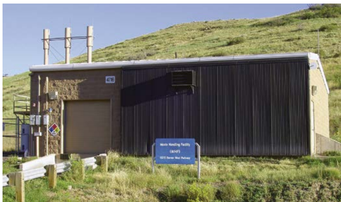
Regulated wastes generated across the STM site are consolidated at the Waste Handling Facility for packaging prior to offsite disposal or recycling. Photo by Sheila Hayter, NREL 14003
