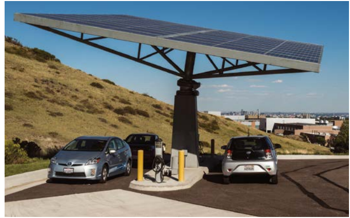
Hybrid electric vehicles charging at the Vehicle Testing and Integration Facility solar canopy. Photo by Dennis Schroeder, NREL 31895
