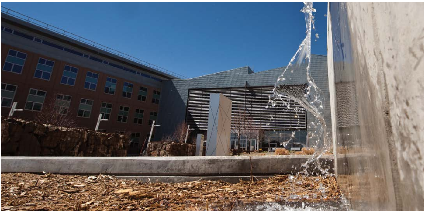
Melting snow from the roof of the Research Support Facility is captured in a landscaped catch basin. These same basins receive stormwater runoff from the roof later in the year, providing water to trees and grasses planted within them. Photo by Dennis Schroeder, NREL 18643
