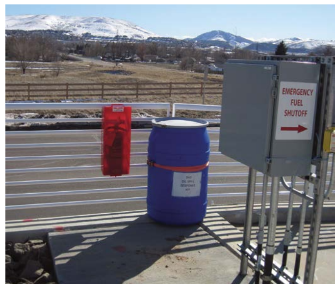
Spill kit near the E-85 tank at the STM site. Photo by Larry Durbin, NREL 36265
