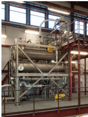
Photo by Dennis Schroeder, NREL/PIX 17684
