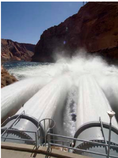
Water being released through river outlet tubes
