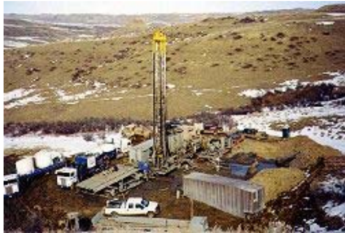
Figure 8 - Photo of Coal Bed Methane Well.
